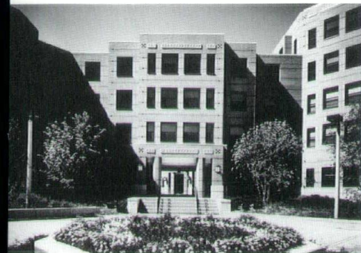
Student Residence & Commons, University of Illinois at Chicago Chicago, Illinois Olomon Cordwell Buenz & Associates, Inc. Photo Steinkamp/Ballogg
