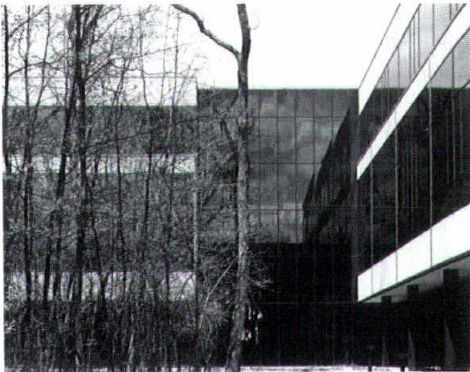
Oakbrook Center Expansion Oak Brook, Illinois Solomon Cordwell Buenz & Associates Photo Don DuBroff, Sadin Photo Group (top)
