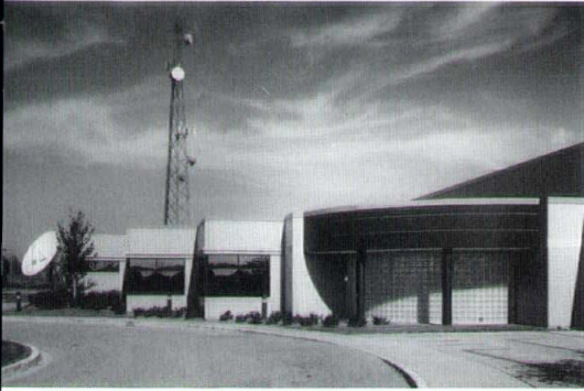
Cellular One Headquarters Deerfield, Illinois Wentkenhoff Saunders Architects, Inc. Photo W. Stephen Saunders (bottom)
