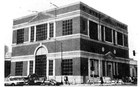
Commonwealth Edison Sub-station, Chicago, IL, Excellence in Masonry '90 Gold Medal winner; Tigerman McCurry, architect; Hansen & Hempel, mason contractor.
