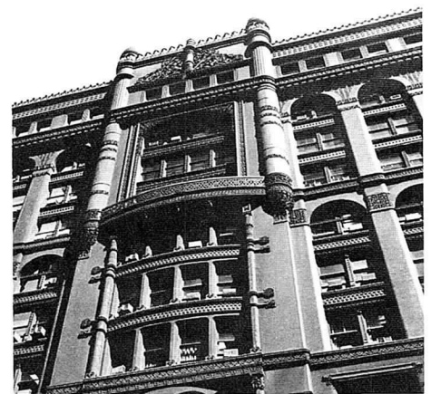
Burnham and Root's Rookery, completed in 1888 and now undergoing restoration, is a feature of the September 22, 1990, Chicago by Design tour. Photo: Richard Nickel for the Commission on Chicago Historical and Architectural Landmarks, courtesy LPCI.
