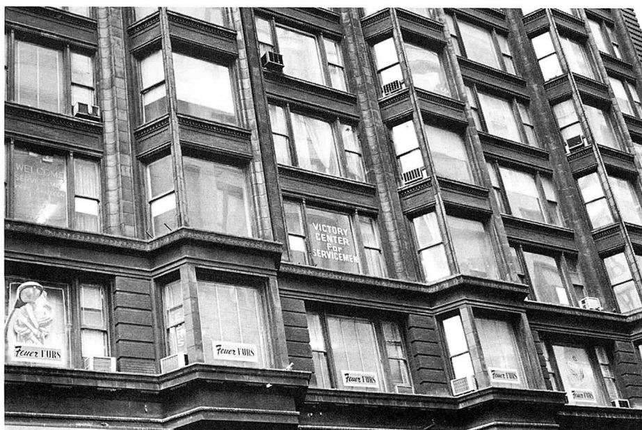
The trend is the destruction of many functional, beautiful urban buildings that have created a unified and vital environment. Will Holabird & Roche' 1904 Chicago Building at State and Madison be next? Photo: courtesy LPCI.
