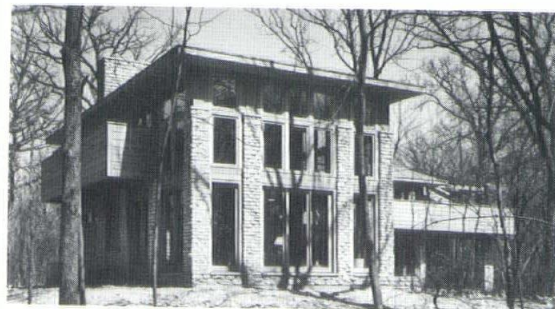
▲ Roth/Wilner House Wayne, Illinois Quinn and Searl, Architects Photo: George Lambros
