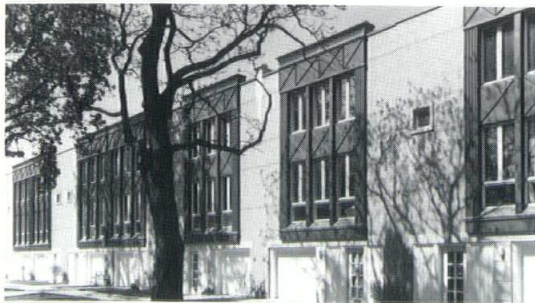
▲ Meyer Residence Chicago, Illinois Peter Landon Architects Ltd. Photo: Ron Gordon
