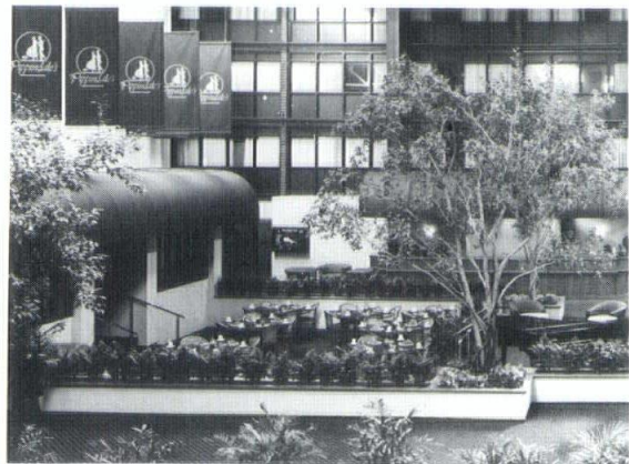
▶ North Shore Holiday Inn Otis Associates, Inc. Photo: Steinkamp/ Ballogg
