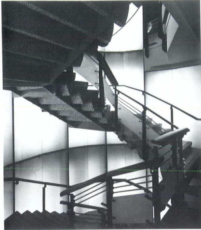
Left: Darcy Bonner, Himmel/Bonner Architects Stanley Korshak at the Crescent, Dallas: terrazzo and steel staircase enclosed by a backlit cylinder of sandblasted glass Photo: R. Greg Hursley
