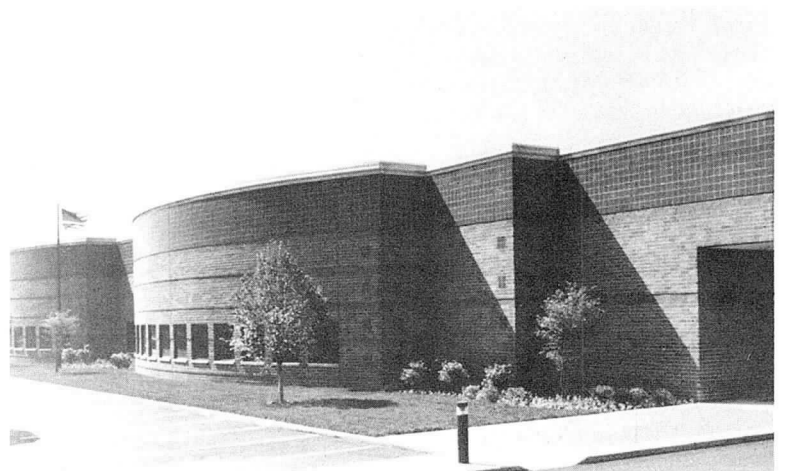
SILVER MEDAL Spiegel Showroom, Greenpoint Building B, Elmhurst, Illinois Architect: Eckenhoff Saunders Architects Mason Contractor: D. H. Johnson Company
