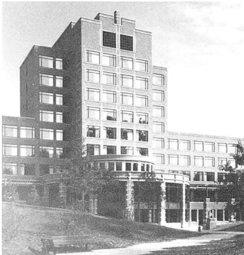
GOLD MEDAL Arthur Anderson & Co. Center for Professional Education, St. Charles Architect: Skidmore, Owings & Merrill Mason Contractor: Crouch-Walker Corporation
