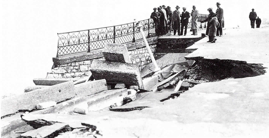
Storm damage in Lincoln Park, Oct. 22-23, 1929.
