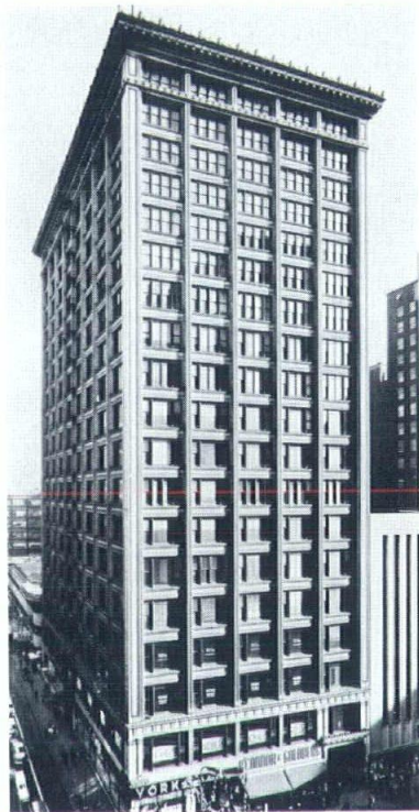
Republic Building Photo: Richard Nickel
