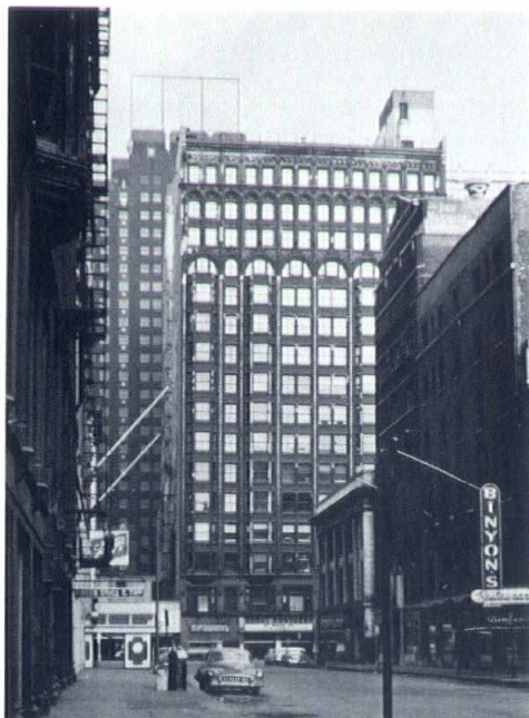
Great Northern Office and Theater Photo: Ben Weese
