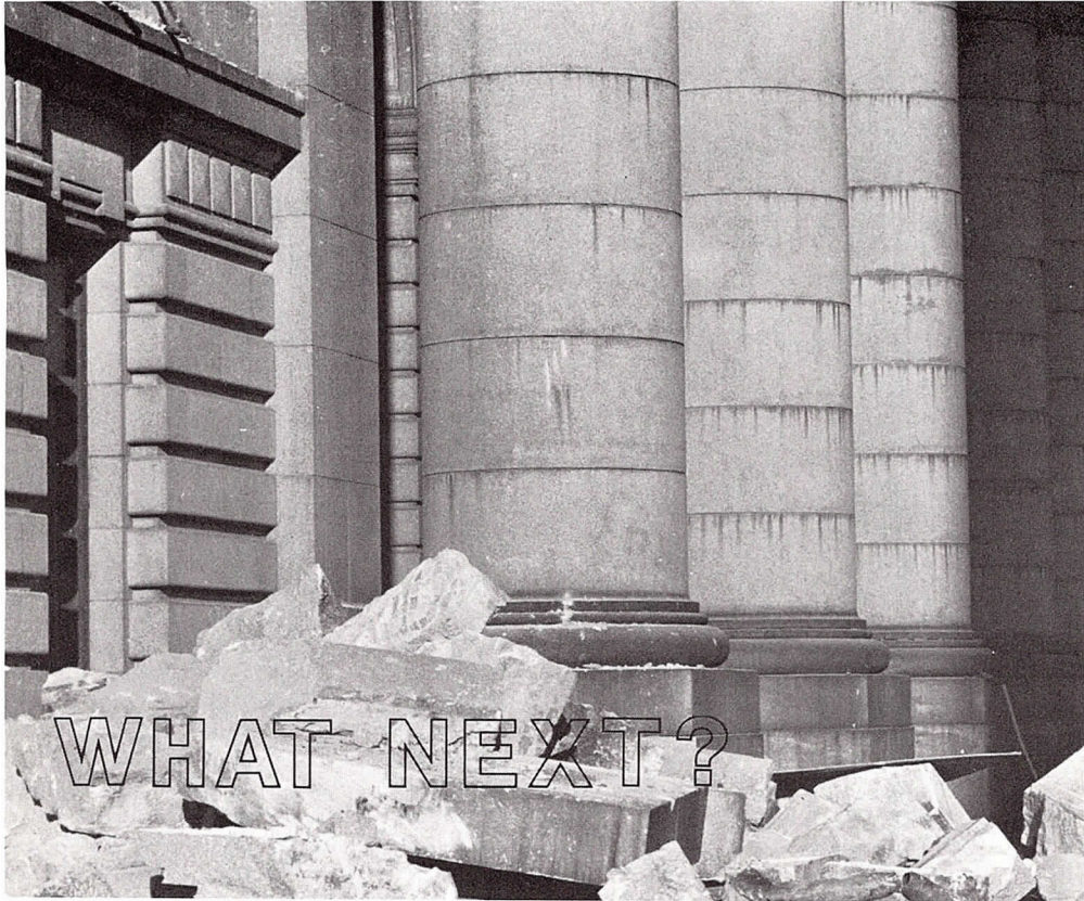
C&W Railway Terminal during September 1984 demolition
