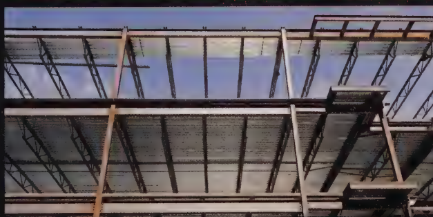
Hambro MD2000 on a conventional structural steel frame
