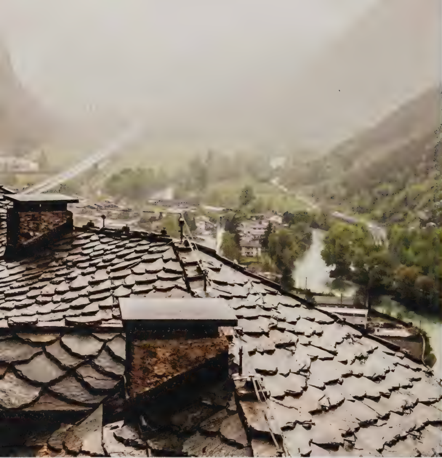
Figure 1 Diamond-shaped slate roof shingles in the Alps are more technically evolved than rectangular shingles because they use the material more efficiently and are more consistently watertight Photo: © iStock.com/koufax73.
