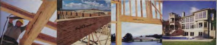
Now a great room can be even greater. With beams, headers, and columns made from Trus Joist Parallam® PSL, you open up a whole new world of opportunities. The superior strength of Parallam PSL is available in lengths up to 60 feet making longer clear spans possible, giving you more design options to offer open, spacious floor plans. Add strength, reliability and design flexibility to your designs with Parallam PSL.
