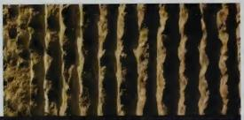
Above: Lindemann Center (Paul Rudolph, 1970). Coarse-aggregate concrete was poured into corrugated formliners and bush-hammered.
