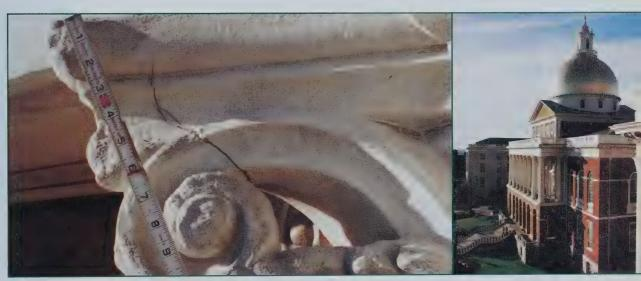
Massachusetts State House, Boston A corner of the addition to the Massachusetts State House, constructed between 1914 and 1917. A ground-based binocular survey of the carved marble cornice, located 90 to 120 feet above grade, did not show serious distress. Subsequent close-up inspection, however, revealed this cracked section, which was removed by simply lifting it away.
