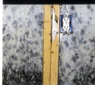
The buyers of these New Hampshire condominiums were stunned to find mold (below) growing inside the firewalls between units only two months after moving in. Delay in closing-in the roof is to blame.
