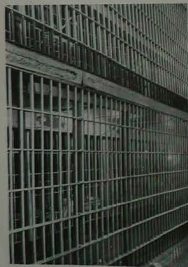
Cell blocks are in poor condition. Note wooden props behind bars to support second tier at weak points. Cracked walls, falling plaster, are common at the prison. Openings under roof in cell block allow birds to enter.
