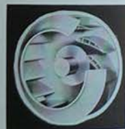
Close-up view of one of the 8 "Chicago" fans ranging in size from 7" to 53". Fans are located in the auditorium building and they move 84,800 cfm.
