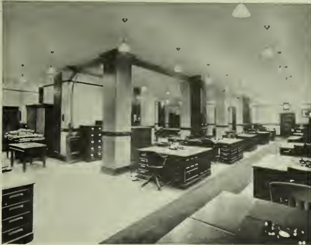
Fig. LXIII. Direct Lighting Installation in Clerical Offices.
