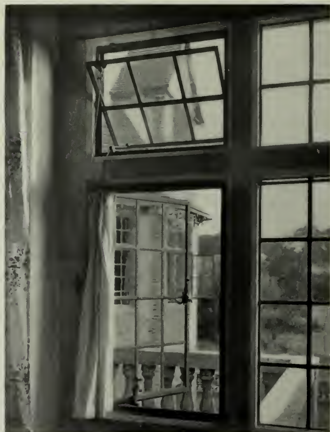
Detail of Metal Casements and Transom Set Within Stone Mullions and Transom Bar
