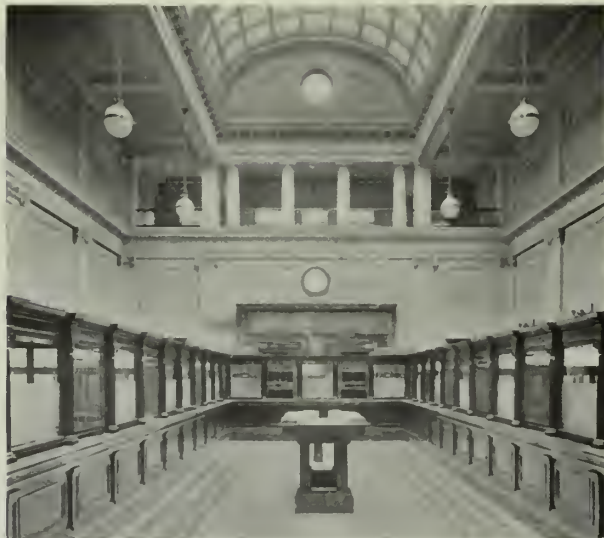
Fig. LXVIII. Direct Lighting from Lamps Enclosed in Prismatic Diffusing Glass Spheres.
