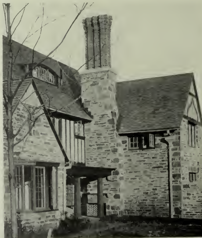
Detail of House at Cynwyd, Pa., Showing Casement Windows Mellor & Meigs, Architects
