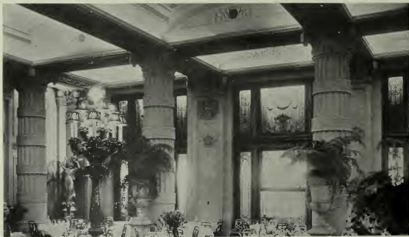
Fig. XXXIX. Palm Room (dining hall), Bellevue-Stratford Hotel, Philadelphia, showing indirect lighting from ceiling coves, supplemented by direct lighting from candelabra on tall floor standards.
