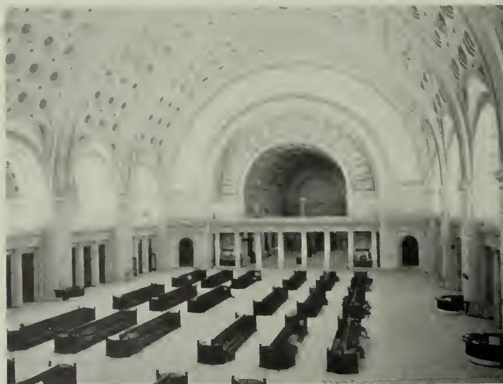
Fig. LIV. Night view of Main Waiting Room, Union Station, Washington, D.C., showing indirect illumination by concealed arc lamps.
