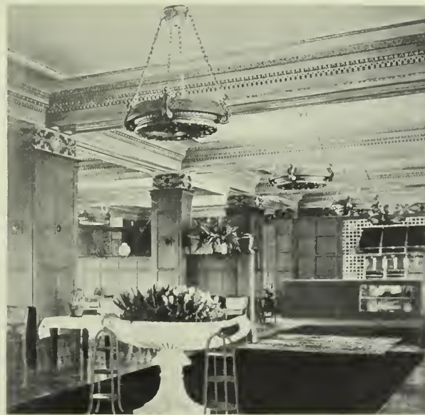
Fig. XLIV. Drawing Room, Whitehall Club, New York City, illuminated by tungsten lamps in opaque (indirect lighting) fixtures.
