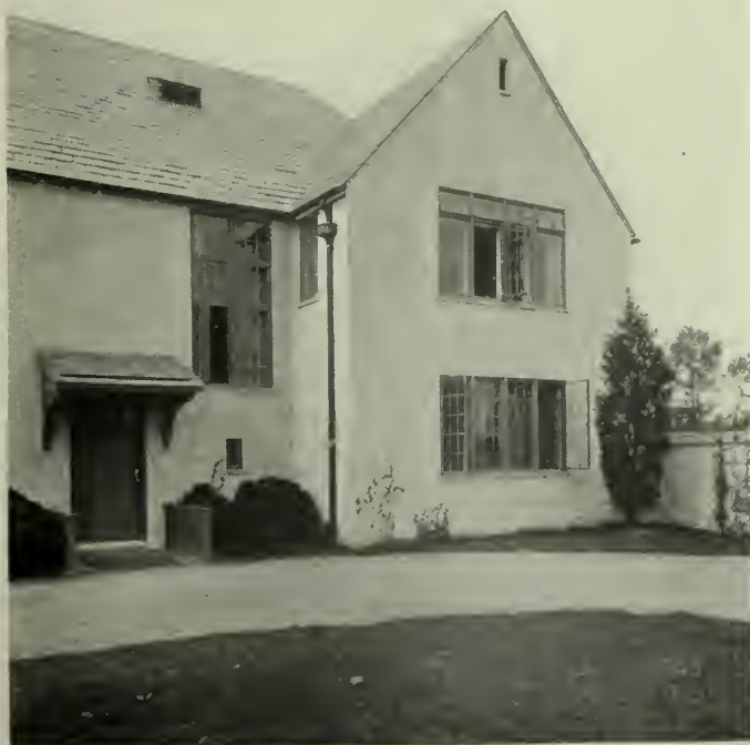
Detail of House at Bernardville, N. J., Showing Metal Casement Windows Delano & Aldrich, Architects
