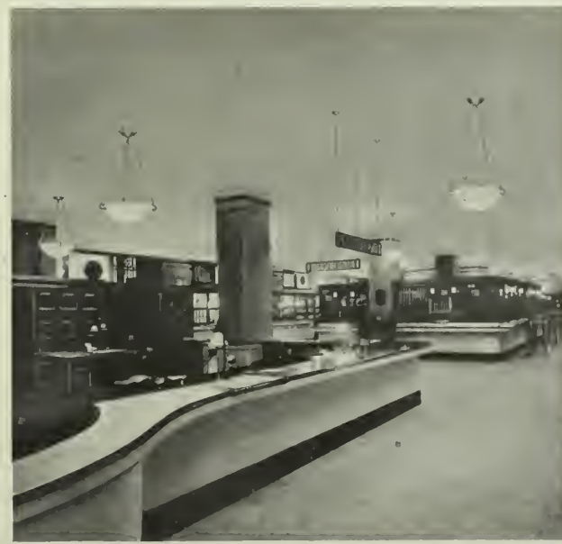
Fig. LXVI. Semi-Indirect Lighting Installation, First National Bank, Chicago, Ill.
