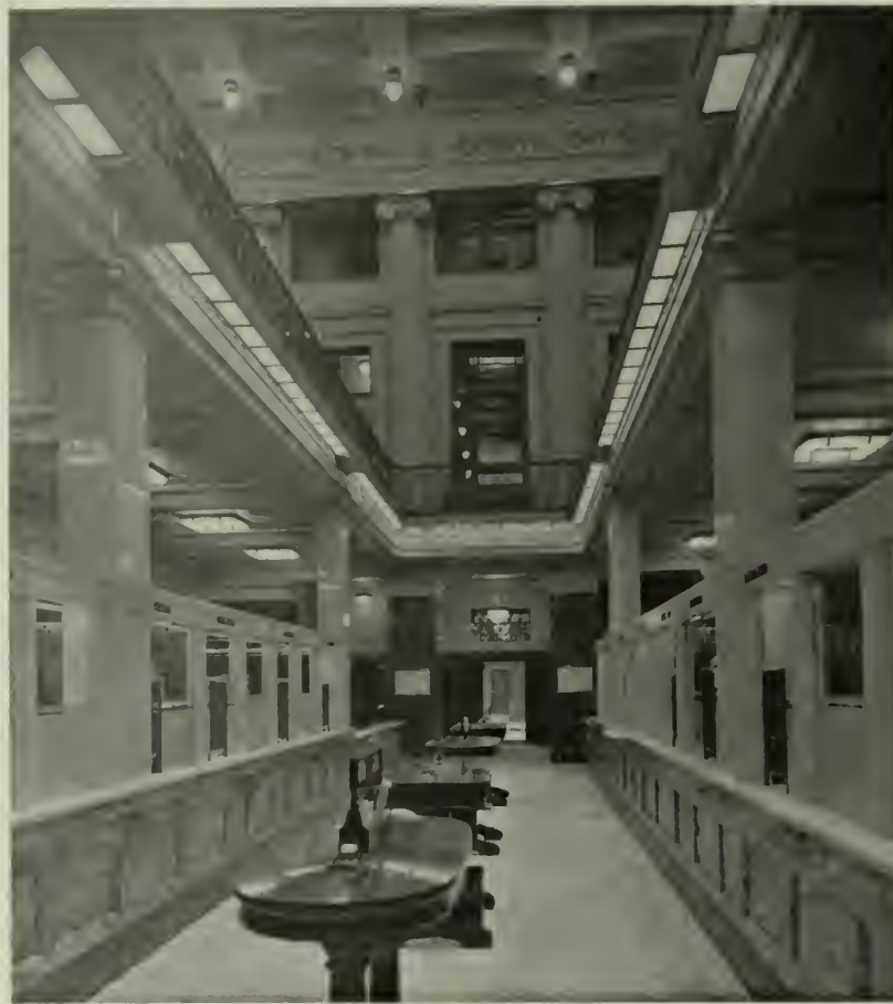
Fig. LXVII. Direct and Semi-Indirect Lighting Installation in Union Trust Company Building, Pittsburgh, Pa.
