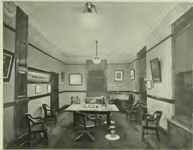
Fig. LXIV. Semi-Indirect Lighting Installation in Private Office.
