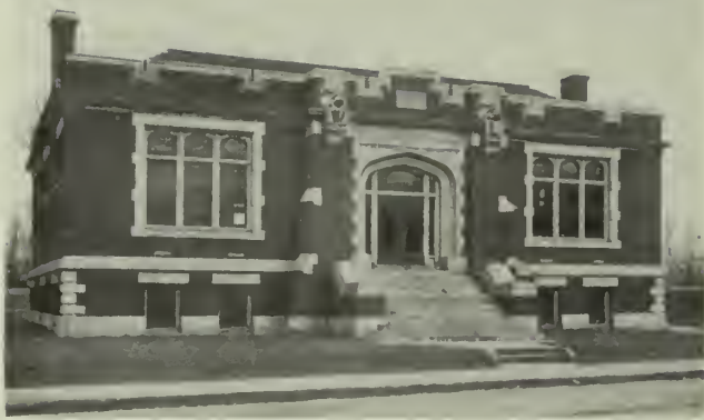
PUBLIC LIBRARY, INDIANAPOLIS, IND. Built of Mosaic Brick-laid Flemish Bond. Made by Western Brick Company. Foltz & Parker, Architects.
