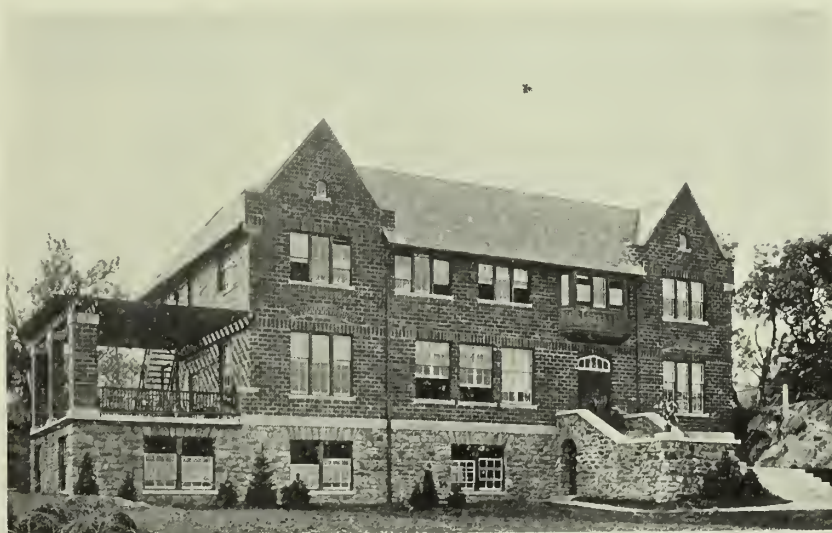
BARNARD SCHOOL, RIVERDALE, N. Y. Built of the new "Tex-Tile," backed with Natco blocks. Mann & McNeille, Architects.
