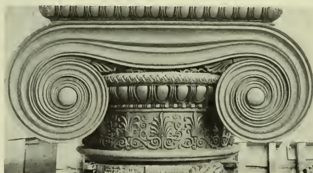
IONIC CAPITAL EIGHT FEET IN WIDTH. Executed by the Atlantic Terra Cotta Company. Garber & Woodward and Tietig & Lee, Architects.
