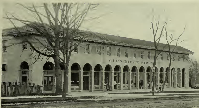
GLEN RIDGE VILLAGE STORES, GLEN RIDGE, N. J. Built of Natco Hollow Tile and faced with brick. Boring & Tilton, Architects.
