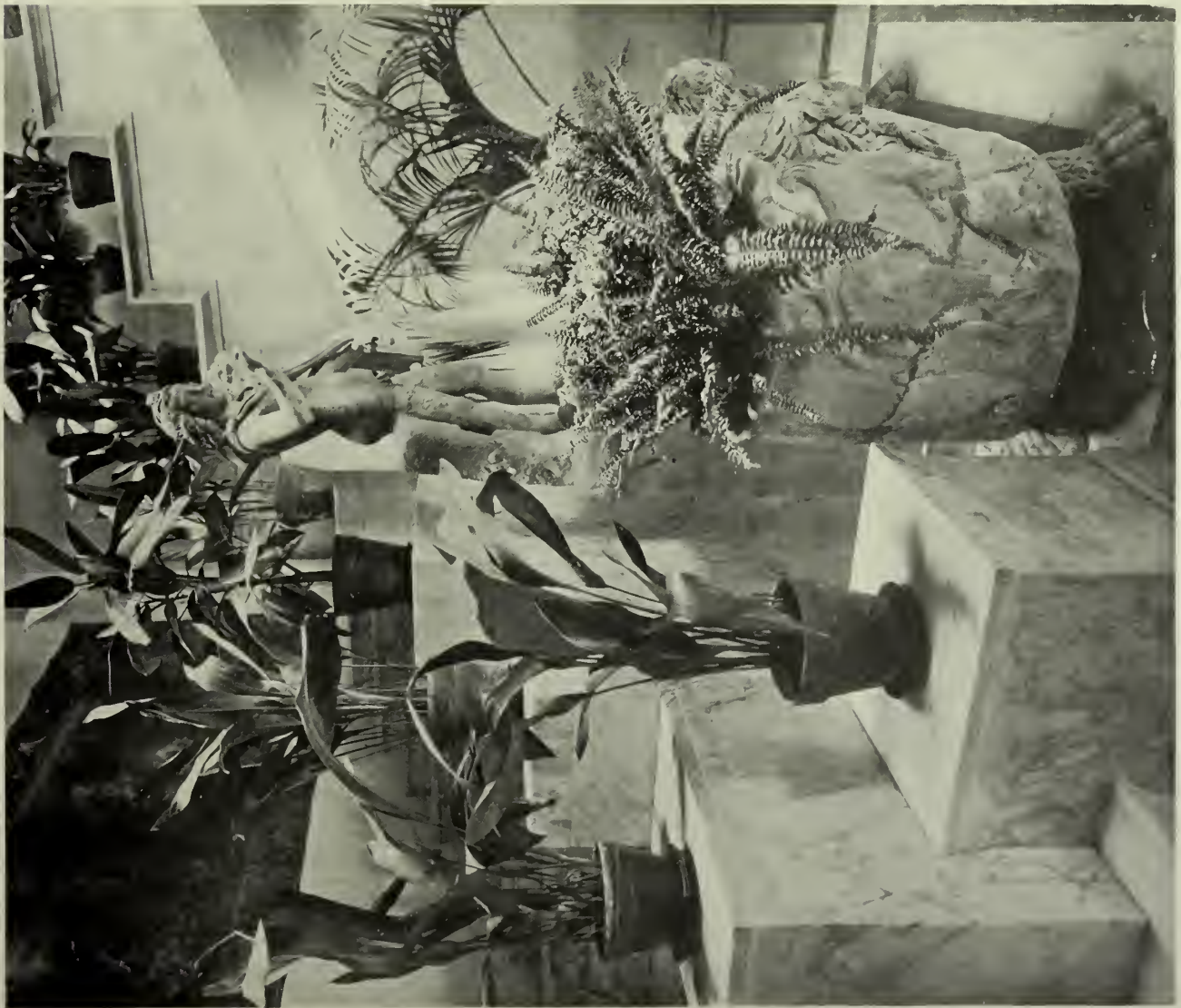
STAIRWAY BY MCKIM, MEAD & WHITE, ARCHITECTS. Great solidity is obtained by this blocky massing of dark veined Pavanazza marble. The barrier of plants serves as a balustrade, the ramp itself being sufficiently wide for the feeling of security.
