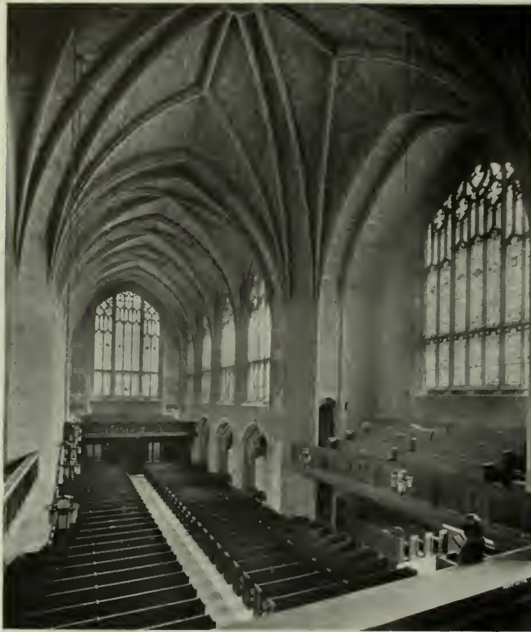
INTERIOR, FIRST BAPTIST CHURCH, PITTSBURGH. Showing Guastavino Tile Ceiling between stone ribs. Cram, Goodhue & Ferguson, Architects.
