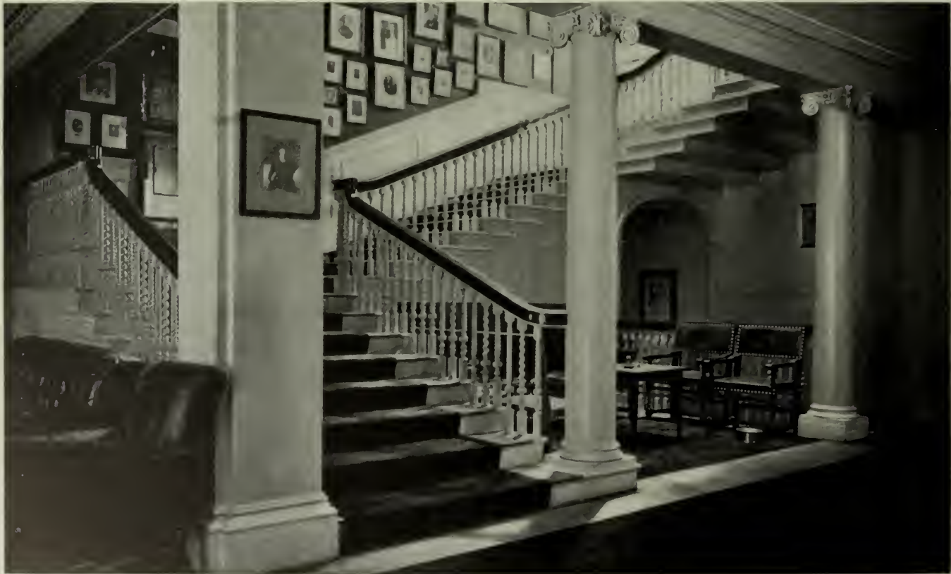
ONE OF MCKIM, MEAD & WHITE'S MOST SUCCESSFUL DOMESTIC STAIRWAYS — HARVARD CLUB, NEW YORK CITY. The ends of the oak treads are painted white to carry the line of the railing. The riser of this stair is 5\frac{3}{4} inches, the tread 14\frac{1}{4} inches, giving a very easy ascent.
