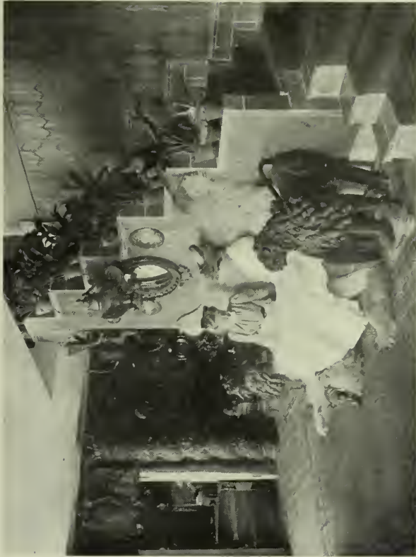
STAIRWAY WITH STEPPED RAMP OF EARLY ORIGIN. The construction is concrete with steps and dado of green tile. The walls are covered with woven bamboo reeds cut from Chinese awnings.
