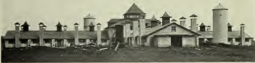
COW BARN, STATE HOSPITAL FOR INSANE, NORRISTOWN, PA. The exterior walls are constructed of 10 inch "Natco" hollow tiles, making a damp-proof, cool-in-summer, warm-in-winter, wall. Baker & Dallett, Architects.
