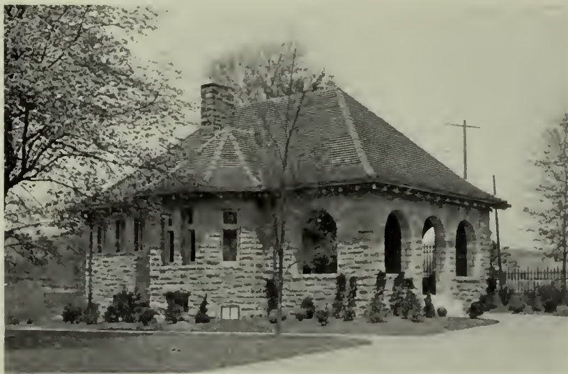
GATE LODGE, SPRING GROVE CEMETERY, CINCINNATI, OHIO. Covered with green glaze "crown" Reinforced English Shingle Tile manufactured by The Cincinnati Roofing Tile & Terra Cotta Company. Elzner & Anderson, Architects.
