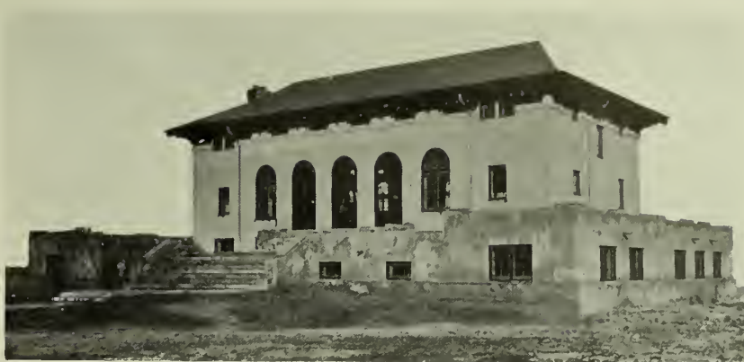
ANNEX TO Y. M. C. A. BUILDING, LEAGUE ISLAND, PHILADELPHIA, PA. Exterior walls constructed of 16 inch "Natco" Hollow Tile and terrace walls of 12 inch "Natco" Hollow Tile, furnished by the National Fire Proofing Company. A. M. Adams, Architect.
