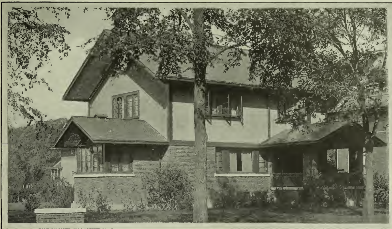
House at River Forest, Ills., designed by William Gray Purcell. The smoking-room is a unique adjunct of the living-room, and with its four double casements is practically a porch in warm weather. The horizontal joints of the brickwork are raked out and the vertical joints struck flush, giving a decided horizontal texture to the first story. The roof is of variegated gray-green and purple slate. The rough cast surfaces above the first story are of a rich warm buff color, with olive green wood trim, and inlays of colored tiles.
