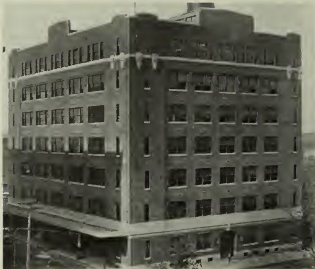
LOOSE-WILES FACTORY, MINNEAPOLIS, MINN. Faced with dark sepia crown tiles, 4 x 12 1/4 inches in size. An example of the interlocking terra cotta facing tile for factory construction made by the Twin City Brick Company. Hewitt & Brown, Architects.
