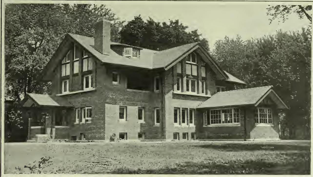
House at Shelbyville, Ill., walls faced with red Danville shale brick in pale red mortar. Roofs, Cloverport shingle tile. Stucco, creamy buff, float finish. Outside rough timber work, etc., stained a warm brown. Terrace and porch floors of Welsh quarry tiles. The boldly projecting living porch connects living and dining room without darkening them. The unusual treatment of the gables avoids the usual baldness of the all brick gable and provides for large windows lighting bedroom, store room, and billiard room.
