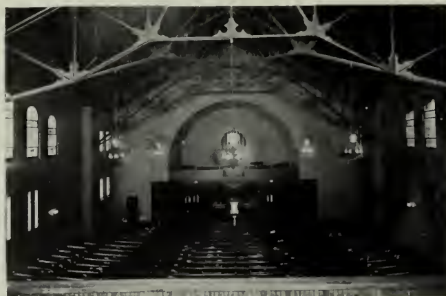
INTERIOR OF BERITH KODESH TEMPLE, ROCHESTER, N. Y. Interior walls faced with Roman brick made by the Ironclay Brick Company. Leon Stern, Architect.
