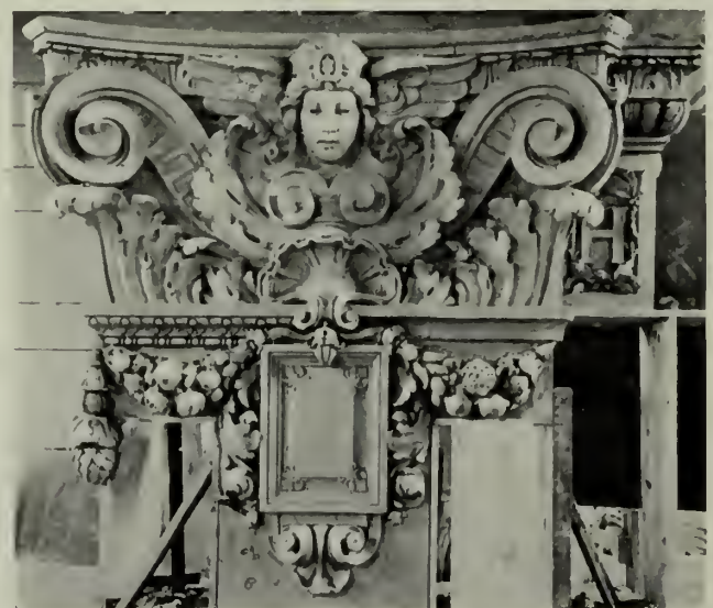
DETAIL FOR HEARST BUILDING. Executed in polychrome enamel terra cotta by Northwestern Terra Cotta Company. James C. Green, Architect.
