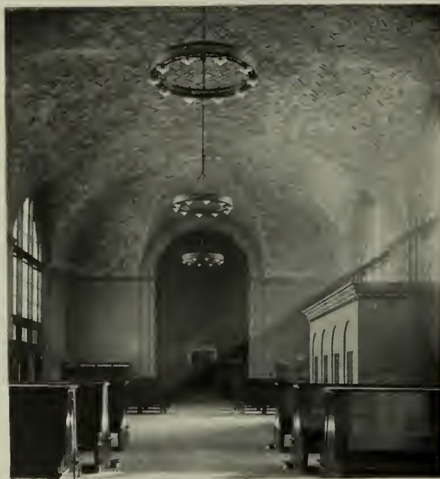
WAITING ROOM, RAILWAY STATION, WATERBURY, CONN. Showing Guastavino ceiling construction. McKim, Mead & White, Architects.
