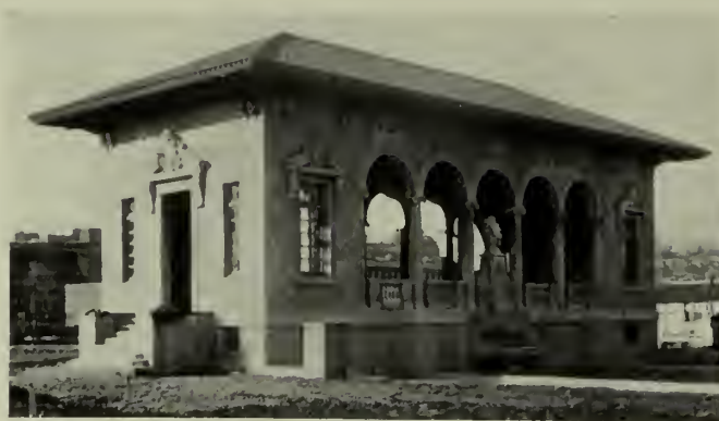
PARK BUILDING, HOBOKEN, N. J. Built of Natco Hollow Tile made by the National Fire Proofing Company. James E. Ware & Son, Architects.
