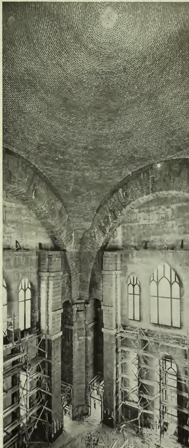
INTERIOR OF DOME, CATHEDRAL OF ST. JOHN THE DIVINE, NEW YORK CITY. Showing dome of Guastavino construction. Heins & LaFarge, Architects.
