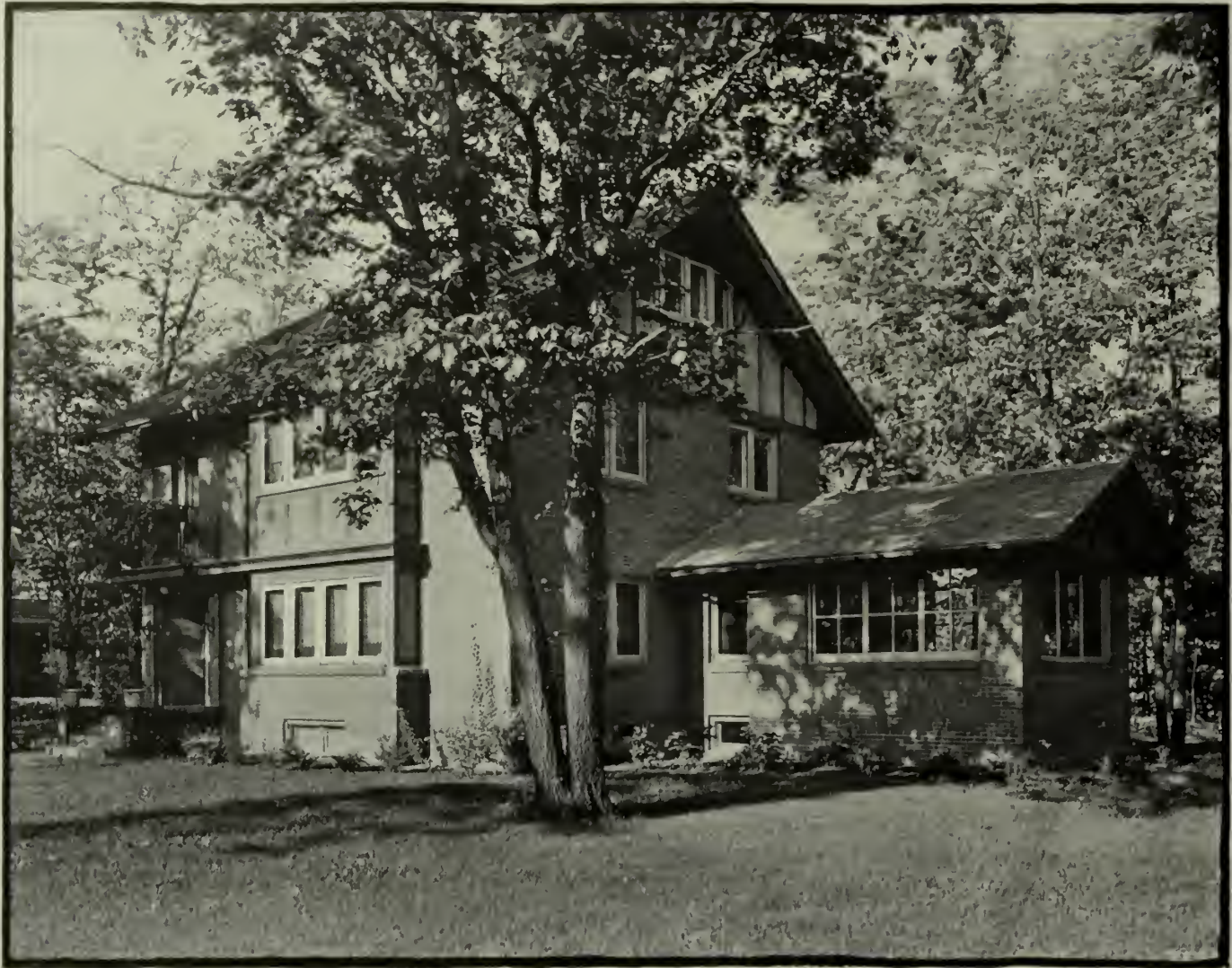
A larger house of the three-bedroom type with roomy attics, stucco and "half timber" treatment of gables, walls of kiln-run pavers, in dull, buff colored mortar. Base, sills, and copings of bricks on edge. Shingled roof. Somewhat unusual in its placing, but very convenient and livable is the large living and dining porch, which is screened in summer and glazed in winter. Cost about $7,500 at Morgan Park, a suburb of Chicago.
