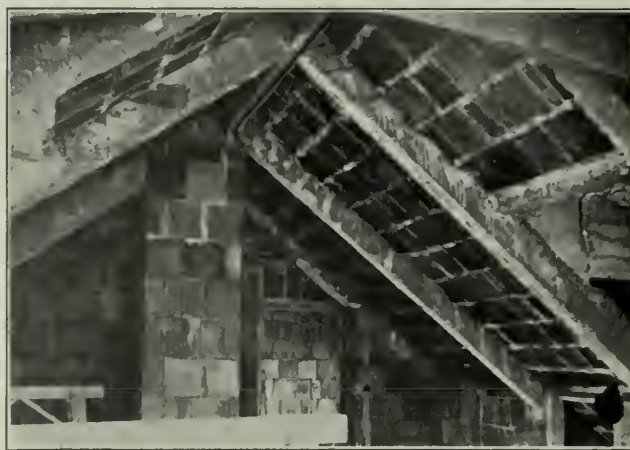
FIG. 11. ROOF BUILT OF BLOCKS WITH REINFORCED CONCRETE RAFTERS.
