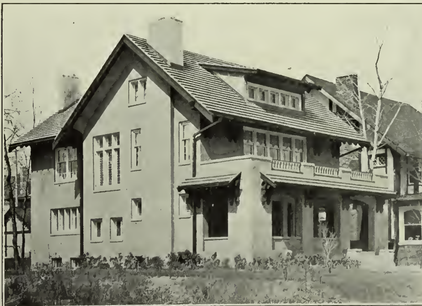
RESIDENCE AT COLUMBUS, OHIO. The green glazed shingle tile were made by the Ludowici-Celadon Company. Frank L. Packard, Architect.
