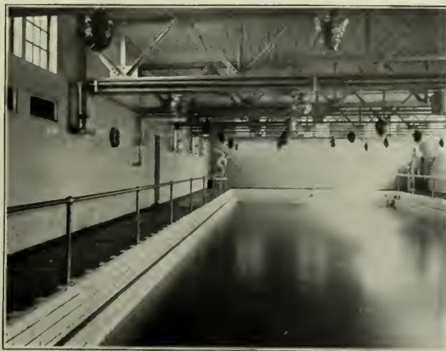
SWIMMING POOL, WORCESTER ACADEMY, WORCESTER, MASS. Showing life rail and gutter built of patented enameled brick, made by American Enameled Brick & Tile Co.
