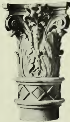
DETAIL BY G. AJELLO, ARCHITECT. Made by New York Architectural Terra Cotta Company.
