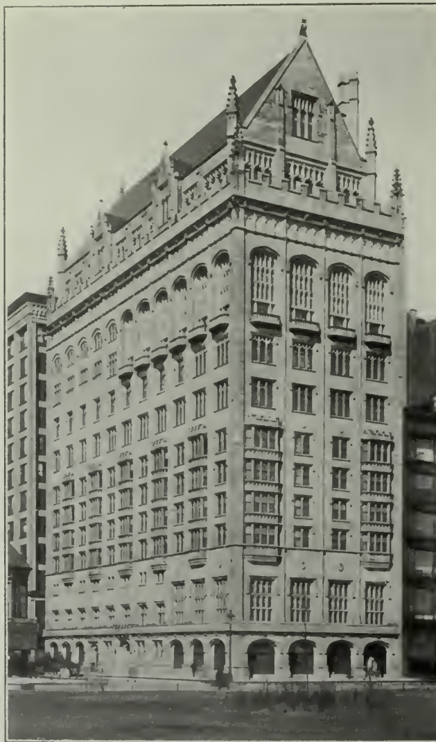
UNIVERSITY CLUB, CHICAGO. Fireproofed throughout with terra cotta hollow tile. Made by National Fire-proofing Company. Holabird & Roche, Architects.
