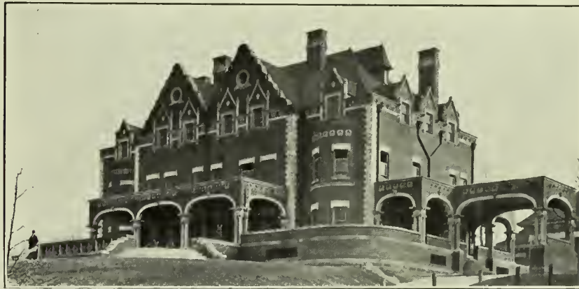
RESIDENCE AT SQUIRREL HILL, PITTSBURG. Built of red roman brick, made by the Bradford Pressed Brick Company.
