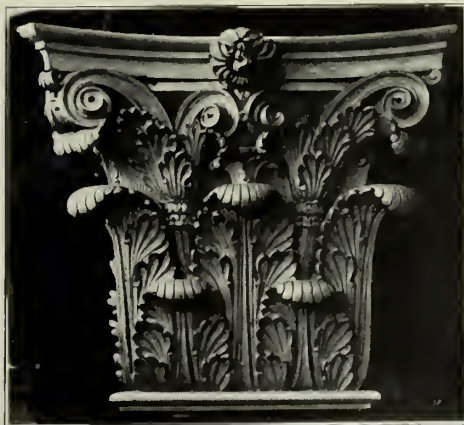
CAPITAL EXECUTED IN TERRA COTTA BY THE NEW JERSEY TERRA COTTA COMPANY. L. Berger & Co., Architects.
