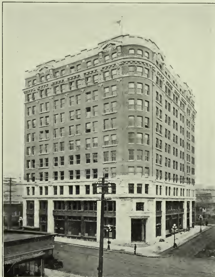
WHITE BUILDING, SEATTLE, WASH. White mat glazed terra cotta, executed by Atlantic Terra Cotta Company. Brick furnished by Hydraulic Pressed Brick Company. Howells & Stokes, Architects.
