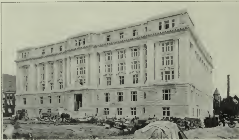
NEW MUNICIPAL BUILDING, WASHINGTON, D. C. Cope & Stewardson, Architects. Fireproofed throughout with Terra Cotta Hollow Tile by National Fireproofing Co.
