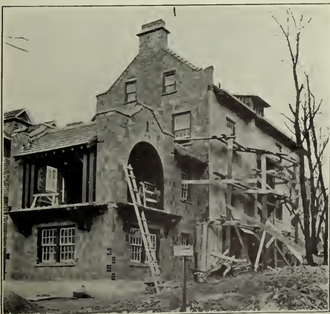
A HOUSE BUILT OF HOLLOW TILE TERRA COTTA BLOCKS WITH EXTERIOR FINISH OF STUCCO.
