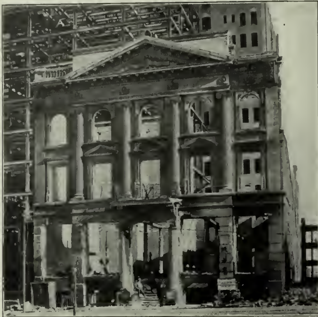
SAN FRANCISCO GAS AND ELECTRIC BLDG. Stone badly spalled, interior completely gutted, but brickwork perfect.
