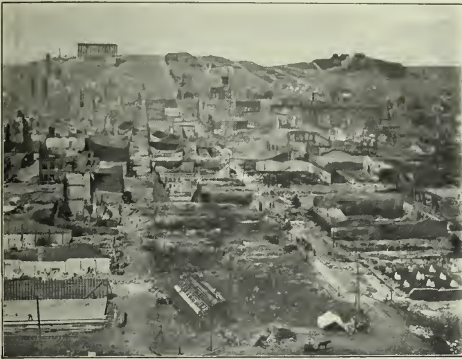
"Fairmont Hotel (exterior walls of terra cotta), though gutted, still crowns Nob Hill, its outer walls practically uninjured, its floors of concrete ruined"
