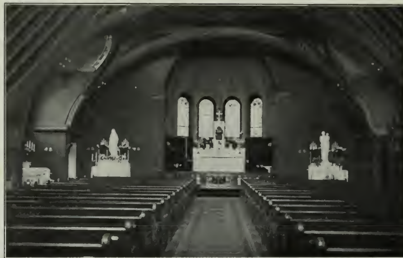
INTERIOR, CHURCH OF OUR LADY OF MT. CARMEL. Example of light, strong and easily built roof truss entirely of planks.
