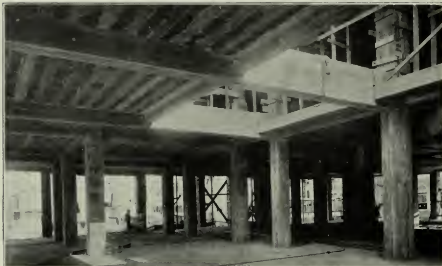
These floors are of varying span between girders according to the exigencies of the plan, and are for spans up to 18 feet. After the wood centering is in place, the tiles, which are 8x8 inches with cross webs, are set end to end in tiers about four inches apart. The reinforcing steel bars are then set between them, and the concrete is tamped into this space.
