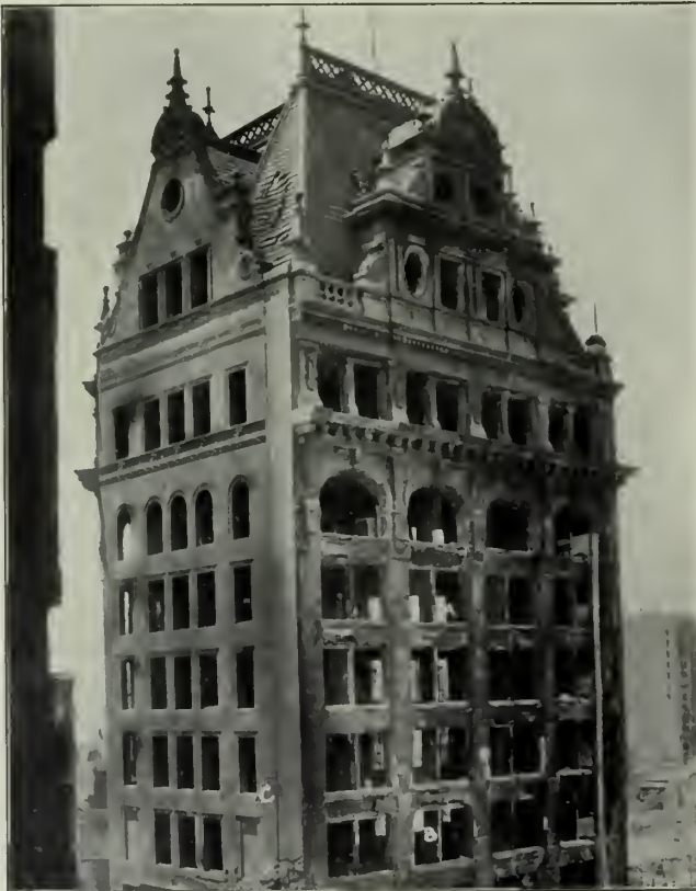
MUTUAL SAVINGS BANK. Stonework A B D destroyed, terra cotta gables above intact.
