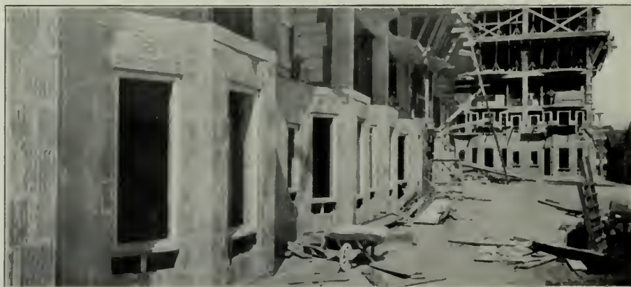
SHOWING EXTERIOR WALLS OF HOLLOW TILES DEEPLY GROOVED TO GIVE A STRONG BOND TO THE PLASTER FINISH.
