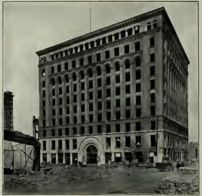
MILLS BUILDING. Stonework A A badly spalled, while the upper eight stories of brick and terra cotta are intact save at a few spots like B.
