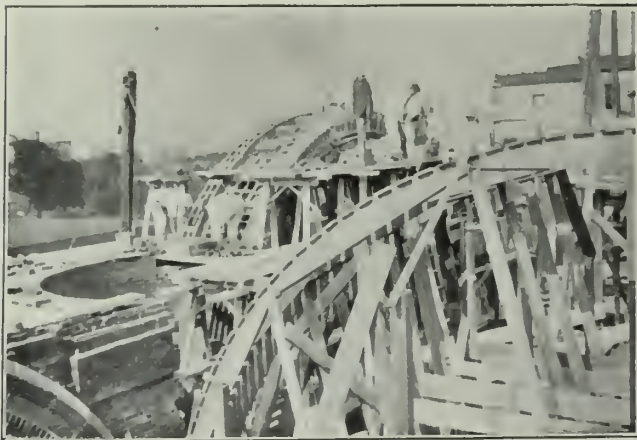
BONDING THE TERRA COTTA BLOCKS WITH THE BRICKWORK OF THE GREAT ARCHES.
