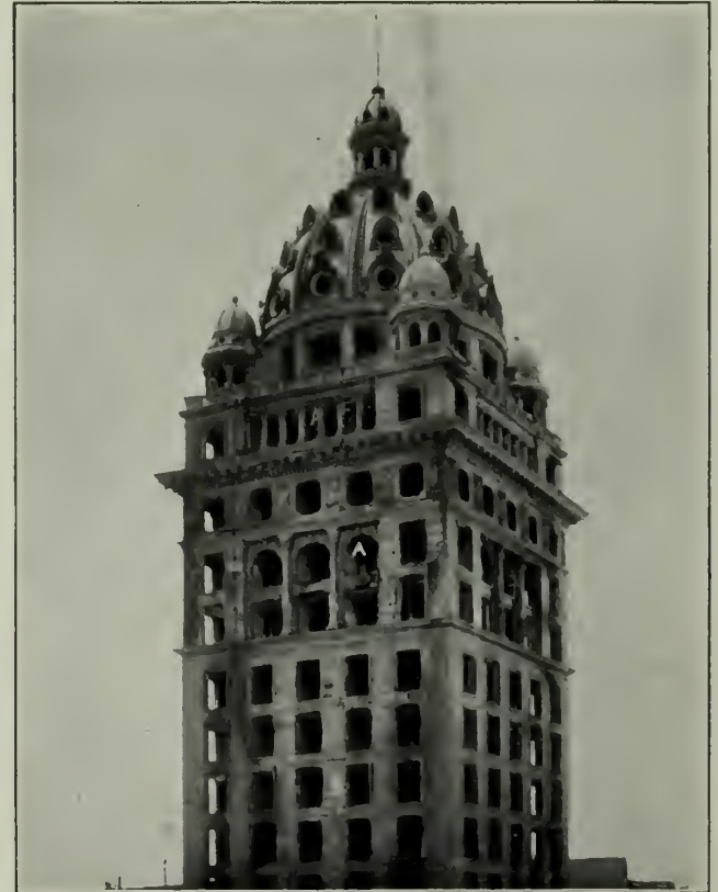
CALL BUILDING. Note effect of fire on stonework at A B, and that terra cotta dome C is undamaged.
