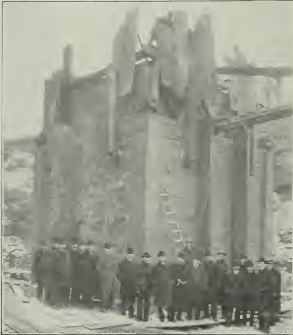
BUILDING BEFORE TEST, LOAD OF 270 POUNDS PER SQUARE FOOT.
