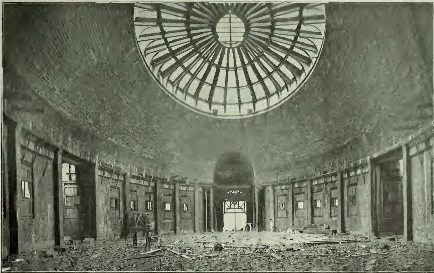
ELLIPTICAL ROTUNDA DOME, NEW YORK CUSTOM HOUSE. Cass Gilbert, Architect. (Span 75 feet by 130 feet. Guastavino construction.)
