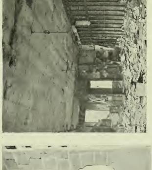
$P_{\rm LATE}$  11.— Methodist Building, eighth floor, showing ceiling of expanded metal and plaster on  $\bf L$  irons and partitions of wooden studs, expanded metal, and plaster.
