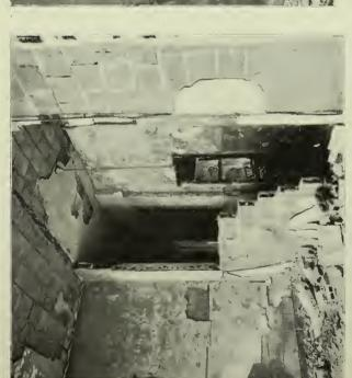
PLATE 10 — Home Office Building, front room in fourth story, showing perfect eiling tiles and damage to partitions caused by use of wooden frames.
