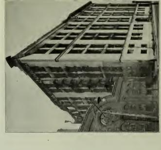
PLATE 5.—Side and rear of Horne Department Store, showing where riveted roof girder pulled out column in rear wall-caused by fall of water tank
