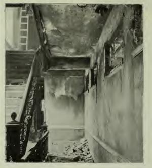
PLATE 13.— Hallway, seventh floor, Methodist Building, showing concrete ceiling and unprotected I beam header warped by heat.
