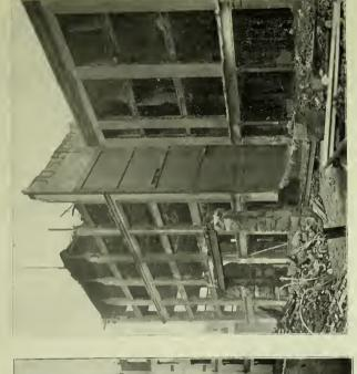
PLATE 9.—Fronts of Horne's Department Store and Horne's Office Building, showing gap made in roof of the former through riveted girder, being pulled down by fall of water tank. Seen over ruins of Jenkins Building.
