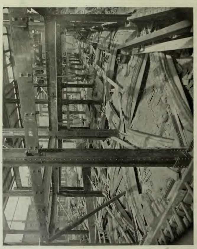
Dome Floor Construction, American Type Foundry Building, Boston. Building, 60 x 180. Seven Floors and Roof.
