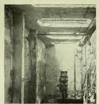
PLATE 12.— Methodist Eufding, seventh noor, showing concrete cening and zo in I beams covered with expanded metal and plaster.
