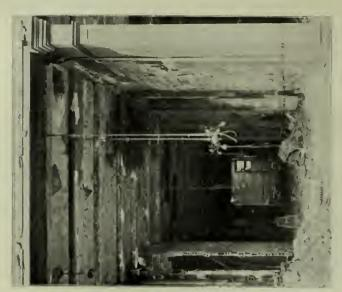
${\rm PLATE}$  6.— West store on Horne Office Building, showing end-pressure hollow-tile floor arches after the fire.
