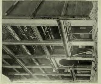
PLATE 3.—Showing front of Horne Department Store and floor arches knocked out through fall of roof, caused by fall of water tank. Beams and girders uninjured except in roof.
