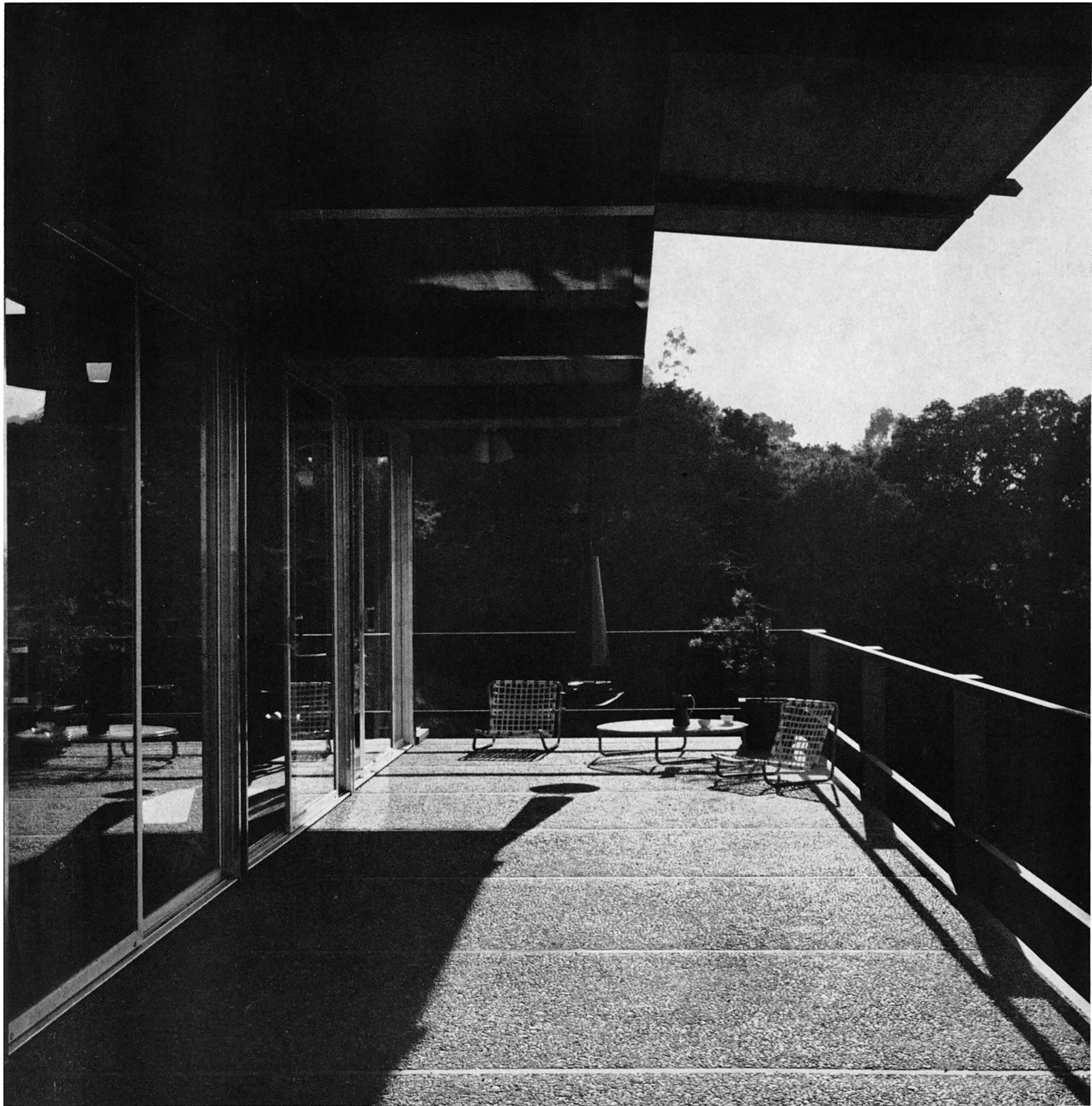
The 10-foot-wide cantilevered deck, overlooking the golf course and the hills beyond, provides 800 square feet of deck, most of it covered. The finish over the exposed concrete aggregate is "Holzite" concrete sealer.
