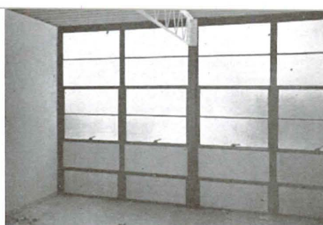
West wall of the storage room and the studio balcony. The obscure glass in the window is Mississippi Glass Company's Focrolite, which is the same as that used in the baths, the front entrance, and the northeast corner of the dining area.
