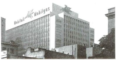
The new building housing the general offices of the General Petroleum Corporation is one of the largest in the Southern California area. The architects have achieved an almost completely fluid floor plan through the use of a 7 foot basic module. This space has thus become almost completely interchangeable through a system of movable partitioning and can be rearranged or readapted as the usefulness of one system is superseded by another.
