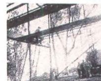
The 11½-ton steel frame shown was erected in a day and a half with a total of 90 man hours.
