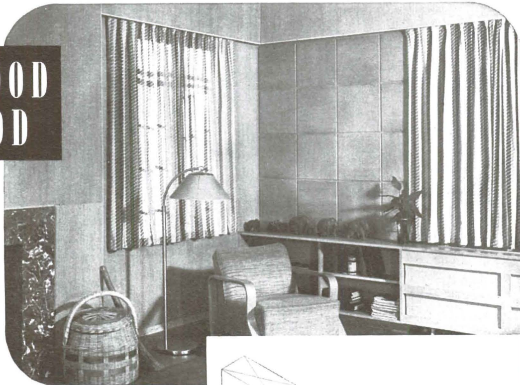
← Showing detail of recessed-joint construction.
