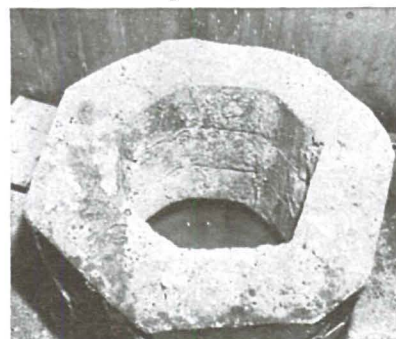
The sump pump well is no longer used. Pump was disconnected months ago. Water still rises to the floor level as can be seen in the above photograph—proving that the floor and walls of the pit are still surrounded by water held back by Aquella.
