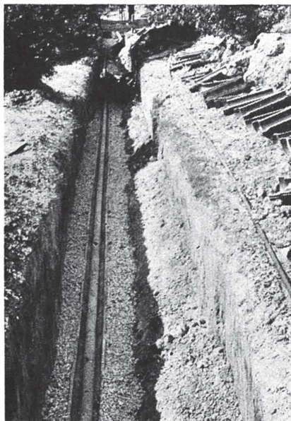
Steam Pipe Line being installed in Ric-wil Tile Conduit at the Citadel.
