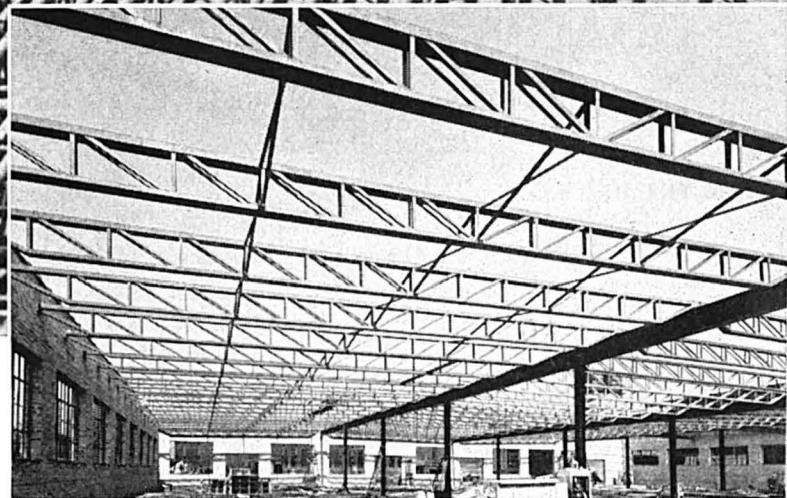
Ceco longspan joists increase floor efficiency by reducing number of columns.
