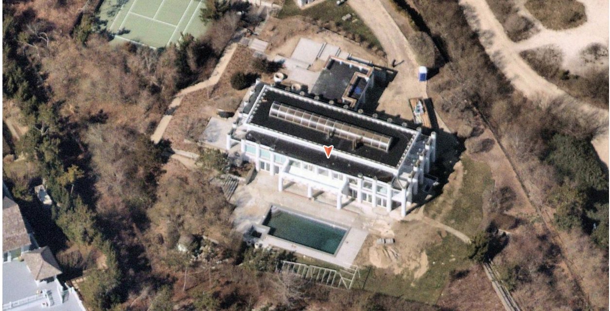
Figure 42. Oblique image of Roslin House at 1880 Meadow Lane, 21 March 2023. Courtesy of the Village of Southampton.
