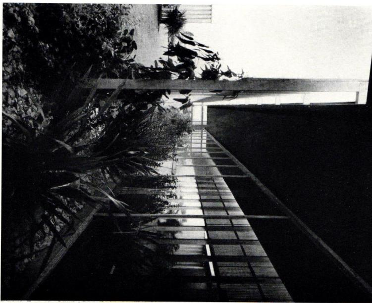
Sunshading devices help reduce the load on the cooling system
