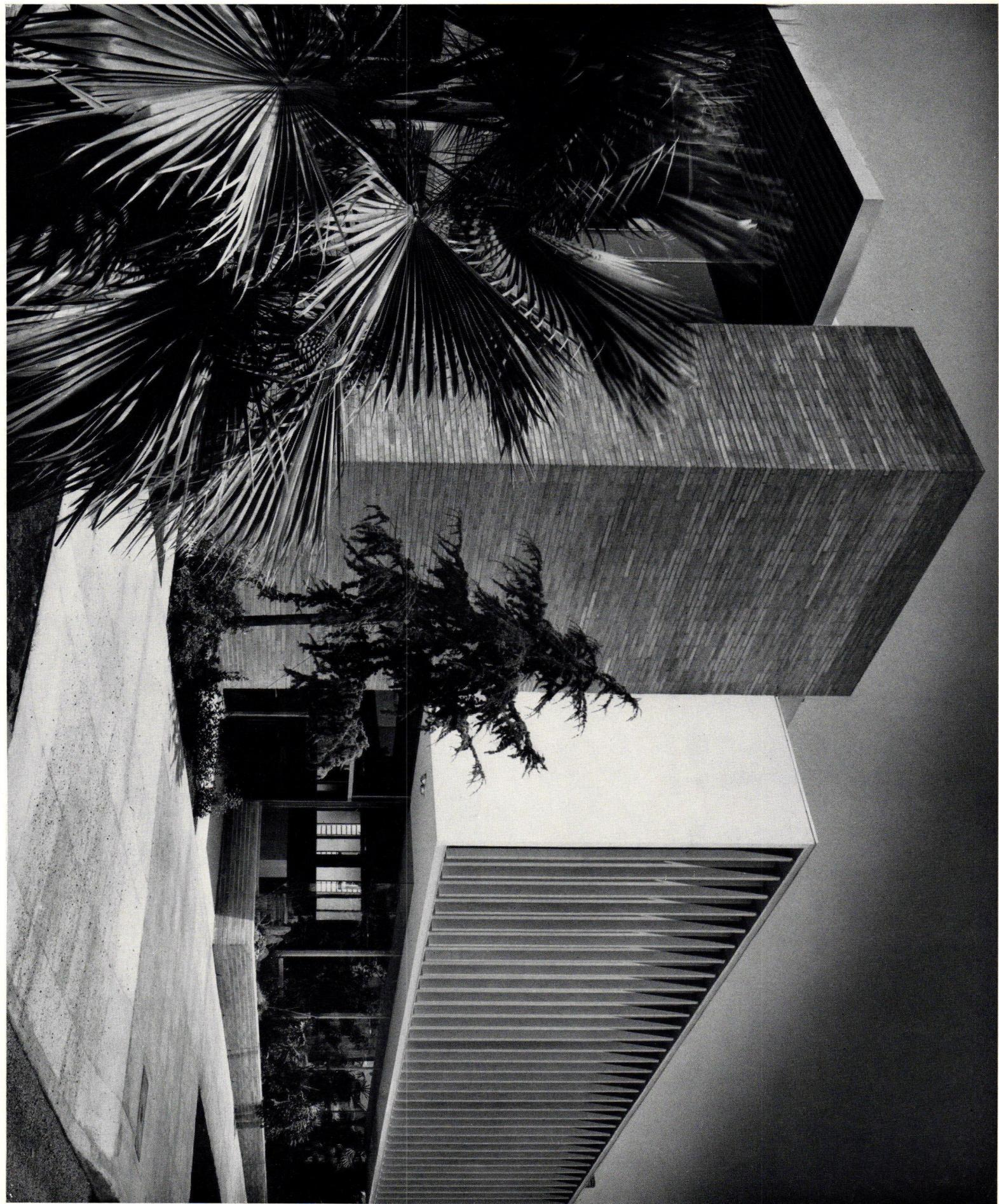
The elevator tower in soft gray brick forms a pleasing contrast to the white plaster, aluminum louvers and plate glass of the street front
