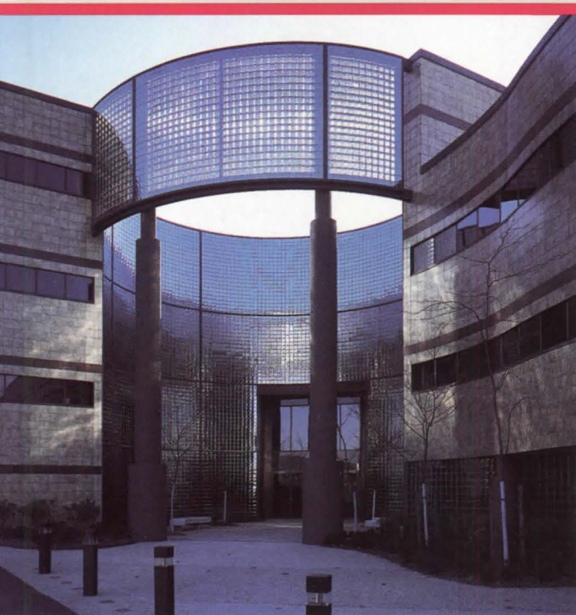
HINES INDUSTRIAL BUILDING Westborough, MA Architect: Drummey Rosanne Anderson, Inc. SOLAR REFLECTIVE Glass Block, VUE® Pattern
