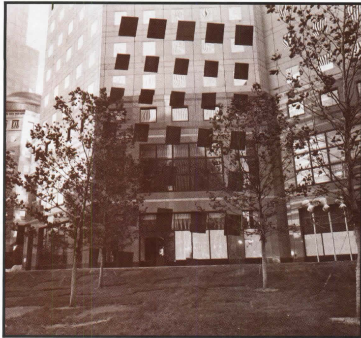
Squares of Battery Park sod climb the walls in Martha Schwartz's installation.
