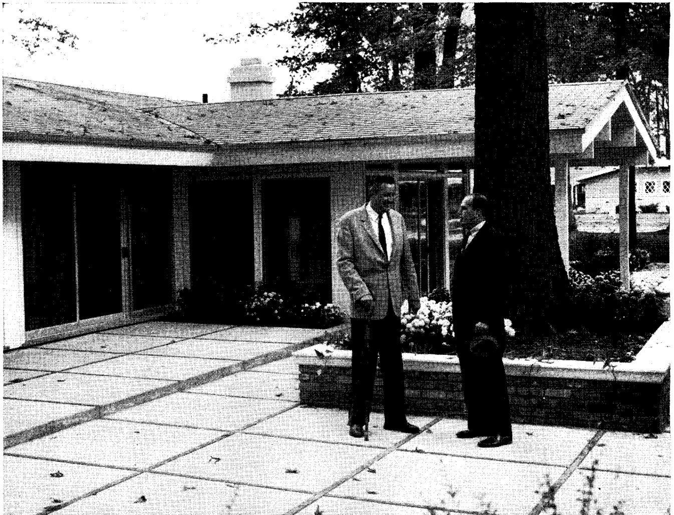
Mr. Scholz (left) at the site of one of his nationally distributed "Mark 58" prefabricated homes with Ken Sprengel of the Telephone Company
