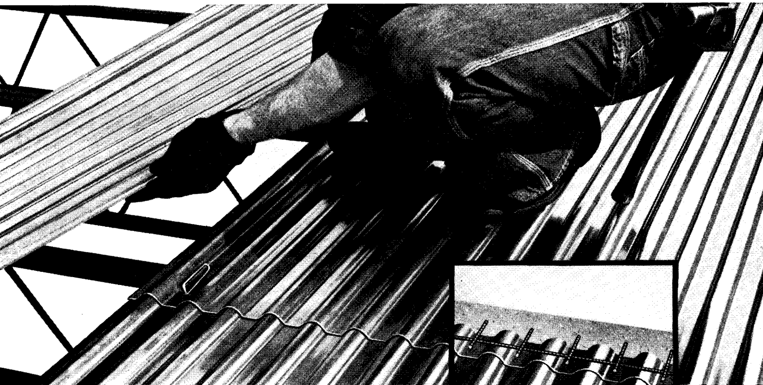
Bethlehem Slabform provides a safe working platform
