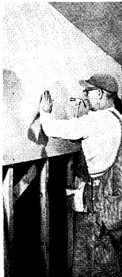
New thermoplastic, elastic flashing (vinylidene chloride copolymer) requires no shop fabrication and is applicable on the job to almost any construction shape or material—including corrugated roofing and siding, vent stacks, and masonry chimneys (above and right). Elasticity prevents breakage of joints or loss of bonding due to movement. Can be cut with knife or heavy-duty scissors. The Dow Chemical Co., Midland, Mich.
