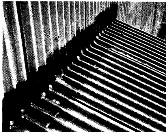
New thermoplastic, elastic flashing (vinylidene chloride copolymer) requires no shop fabrication and is applicable on the job to almost any construction shape or material—including corrugated roofing and siding, vent stacks, and masonry chimneys (above and right). Elasticity prevents breakage of joints or loss of bonding due to movement. Can be cut with knife or heavy-duty scissors. The Dow Chemical Co., Midland, Mich.
