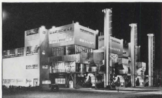
"C" Panel Walls of The Kansas Power and Light Company, Hutchinson. Both steel and aluminum and "combination" panels were used. Architect: Black & Veatch, Kansas City.
