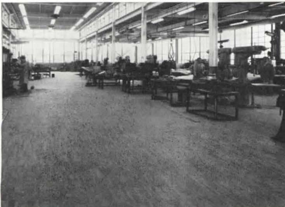
Floor of patterned Northern Hard Maple in Koppy Tool & Die plant, Ferndale, Mich. Campbell Const. Co., Gen'l Contractors.
