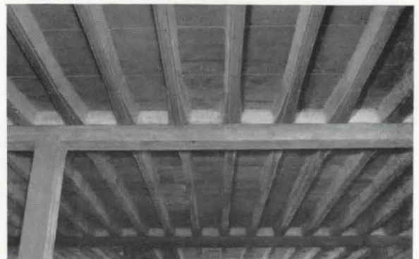
CONCRETE JOISTS eliminate much of the concrete below the neutral axis, saving money, saving material. Suited to buildings with long spans: stores, offices, apartments, hotels.
