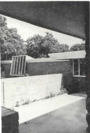
Below—exterior and interior of the weaving studio, with its generous north skylight.
