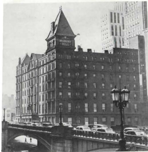
The old Murray Hill Hotel — site of 100 Park Avenue — where there were months of legal battles before the last guests finally moved.
