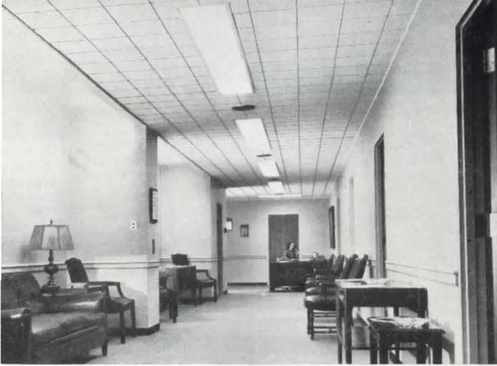
and below: Installation in American Airlines, Inc., Offices. Architect: Kahn Acoustical Contractor: National Acoustics Co., N.Y.C.
