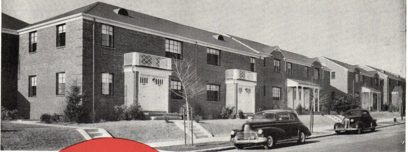
Units of a 576-family housing development equipped with B & G Hydro-Flo Heating.
