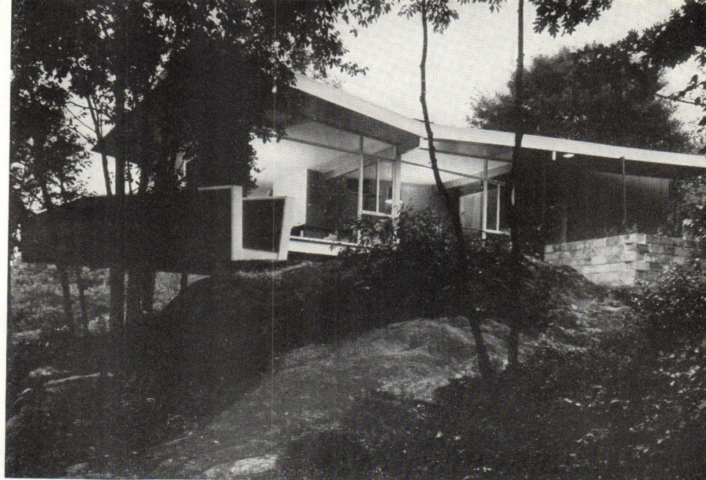
Right: view of southwest corner of house, showing return of ramp from sun deck to top of rock outcropping.
