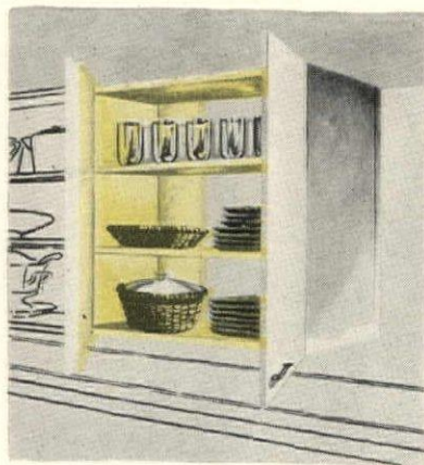
DIVIDER WALL UNIT makes it possible to open cabinet from both sides, saves steps.
