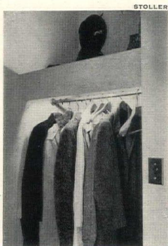
CLOSET LIGHTING by concealed fluorescent strip does two jobs at once. Clothing hung on racks can be easily identified. Hats are kept on shelf above.
