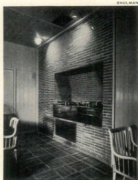
BARBECUE built into a dining room wall has a hot plate at left, sink in the center, grill at right. Fan eliminates cooking odors.
