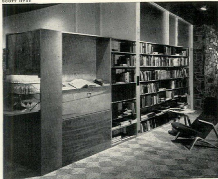
STORAGE WALL separates living and dining rooms. On the living room side, it is a reading wall with special shelves and a slanted surface for using bulky reference books. Built under the reading niche is a drop-leaf desk. A cabinet at the free end holds wine glasses and decanters; its hinged fold-up door is used as a drop-leaf serving table. Concealed light tubes in the center cabinet set off the crystal.
