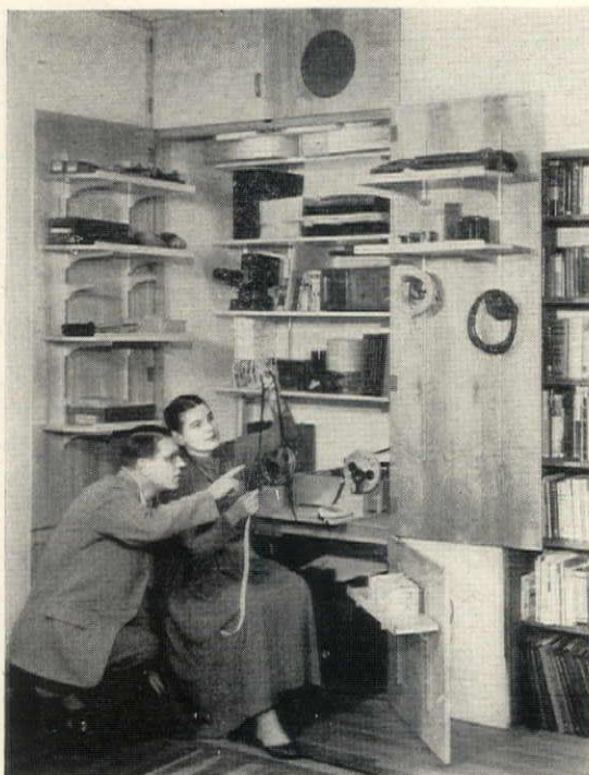
HOLD-ALL CUPBOARD which the Hoskens built alongside living room bookcase and fireplace. They capitalized on its depth by cantilevering shelves inside flush plywood doors. Loudspeaker of phonograph is above doors. Above, the closet doors closed; left, doors open.
