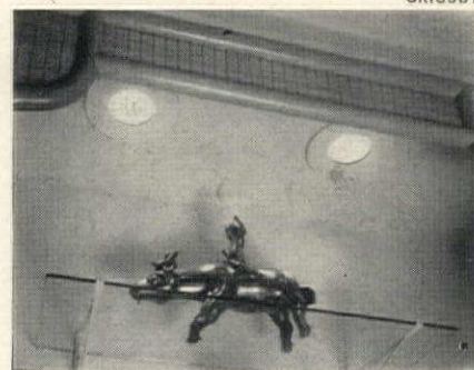
GLARELESS LIGHT OVER MIRROR by use of new glass lens. Pebble texture kills all shadows, black enameled ridges kill glare. Light is diffused and tinted.
