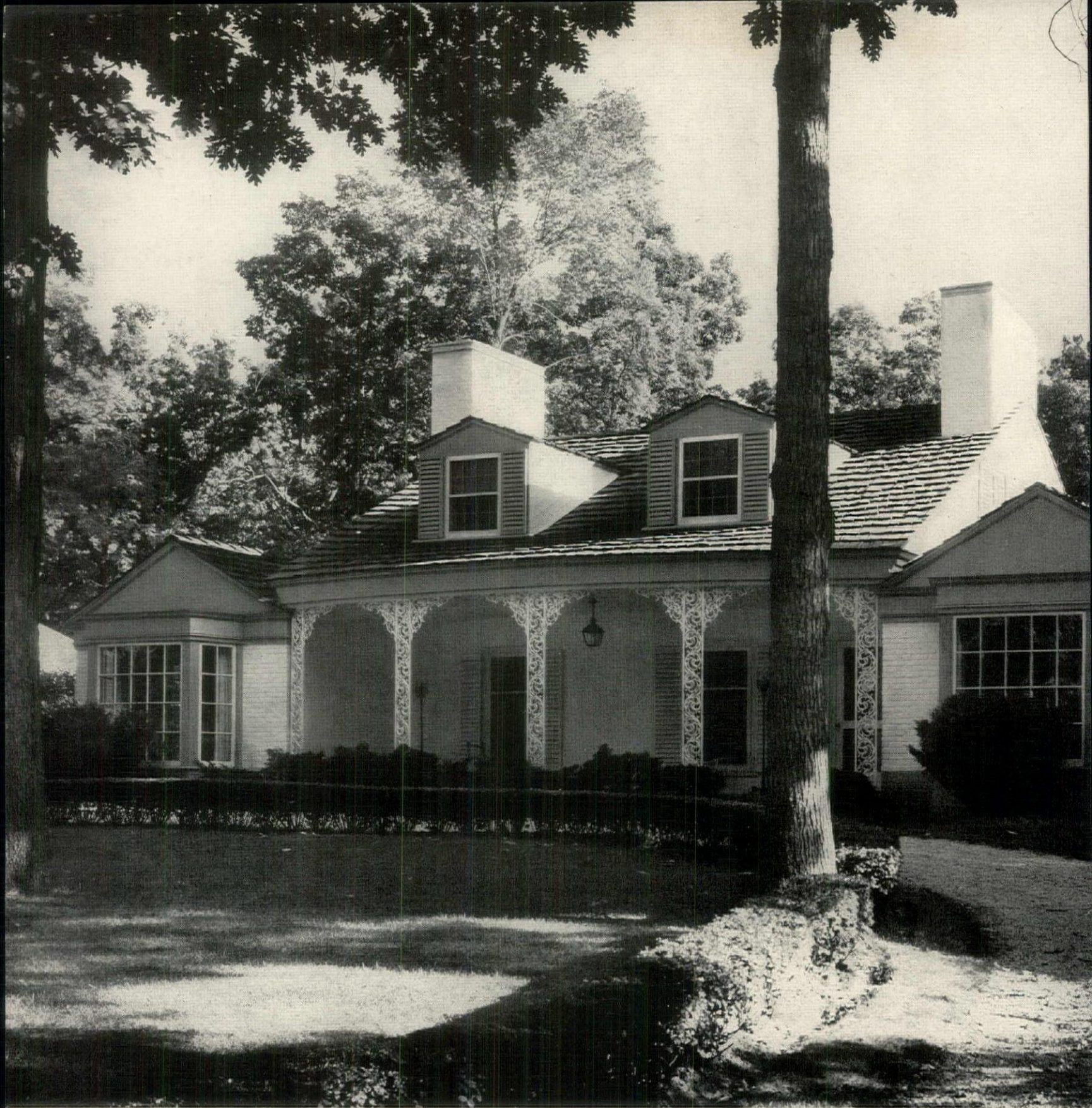
THE BOW-SHAPED PORCH across the house is framed in delicate wrought iron, painted straw yellow like the brick walls. All other trim is French gray.
