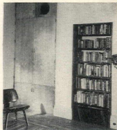
HOLD-ALL CUPBOARD which the Hoskens built alongside living room bookcase and fireplace. They capitalized on its depth by cantilevering shelves inside flush plywood doors. Loudspeaker of phonograph is above doors. Above, the closet doors closed; left, doors open.
