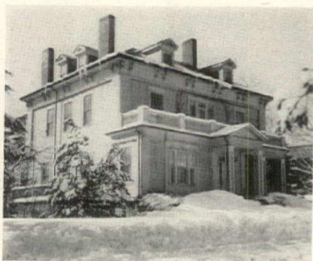
HOSKENS have balcony floor in old house
