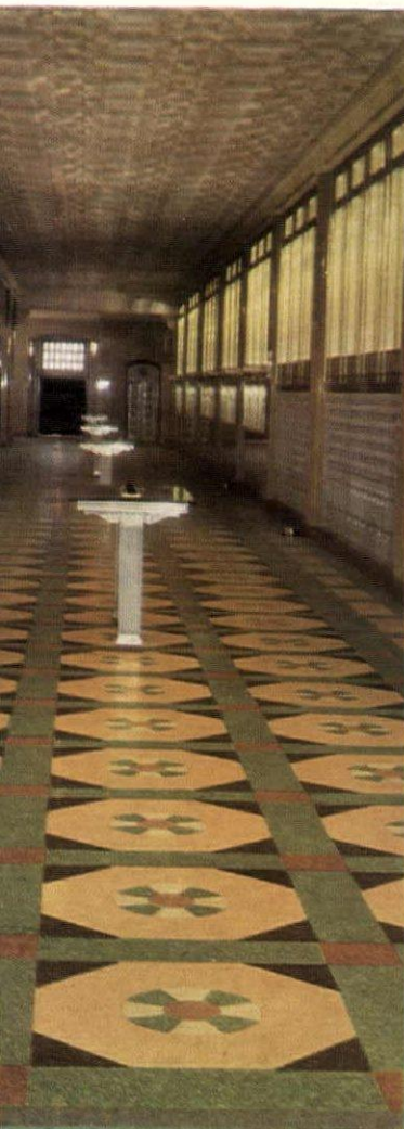
TERRAZZO floor, made with Atlas White cement, withstands daily traffic in Sacramento, Cal., Post Office. Architects, Starks and Anderson, Sacramento; Contractor, California Terrazzo Marble Co., San Francisco.
