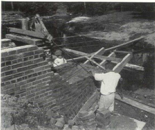
ALL-BRICK bridge, recently built on the grounds of the Melrose Country Club, near Philadelphia. Here reinforcing rods were placed in the upper part of the arch so as to permit its construction on the cantilever principle with simple movable centering supported by the arch itself. Platform is built from 3¾ in. precast, cantilever brick slabs, stiffened at the edge with a brick curb. Precast slabs of this type are being used in the mid-West for porch and terrace floors, eliminating the need for cinder fill and separate supporting slabs for brick pavement.
