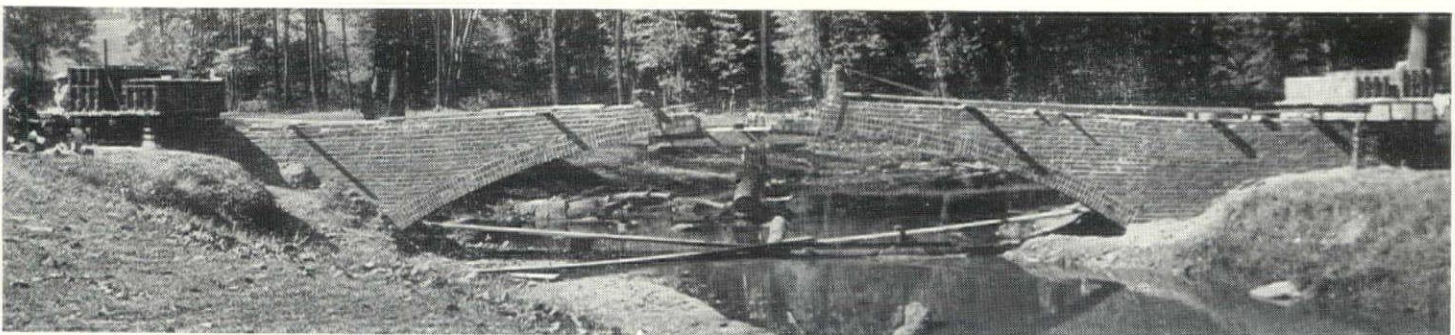
ALL-BRICK bridge, recently built on the grounds of the Melrose Country Club, near Philadelphia. Here reinforcing rods were placed in the upper part of the arch so as to permit its construction on the cantilever principle with simple movable centering supported by the arch itself. Platform is built from 3¾ in. precast, cantilever brick slabs, stiffened at the edge with a brick curb. Precast slabs of this type are being used in the mid-West for porch and terrace floors, eliminating the need for cinder fill and separate supporting slabs for brick pavement.
