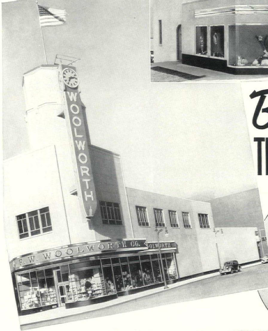
Woolworth's — Brasco Stainless Steel Store Front Construction, entrance doors, canopies. Arch., George Braun, Jr.; Superintendent of Const., E. H. Anderson, both of Chicago.
