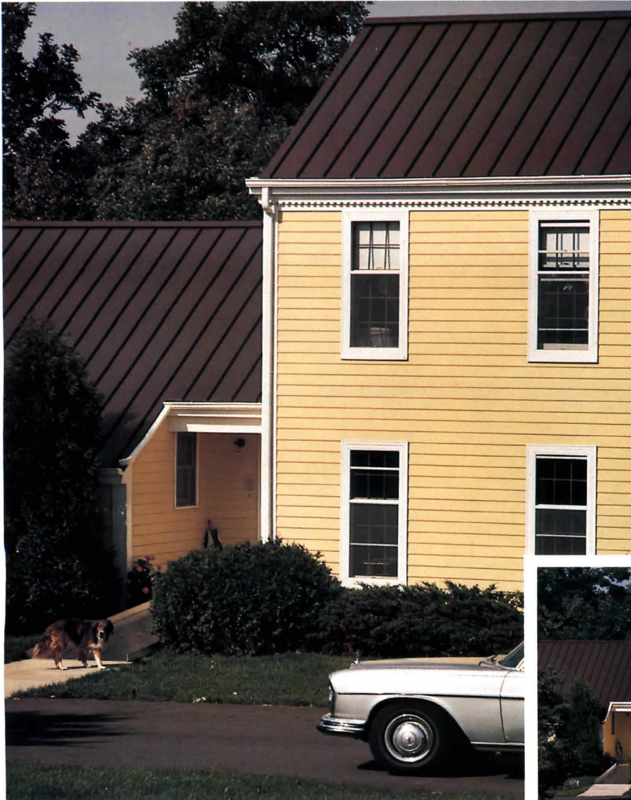
Sheet metal contractor - John A. Dalsin & Son, Minneapolis, Minnesota.
