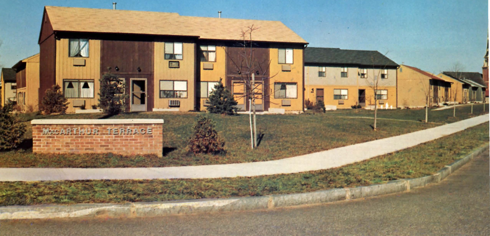
MacArthur Terrace, Chicopee, Massachusetts/A HUD 236 Project for Chicopee Housing Associates/Architect—Reinhardt Associates, Inc./General Contractor—Dimeo Construction
