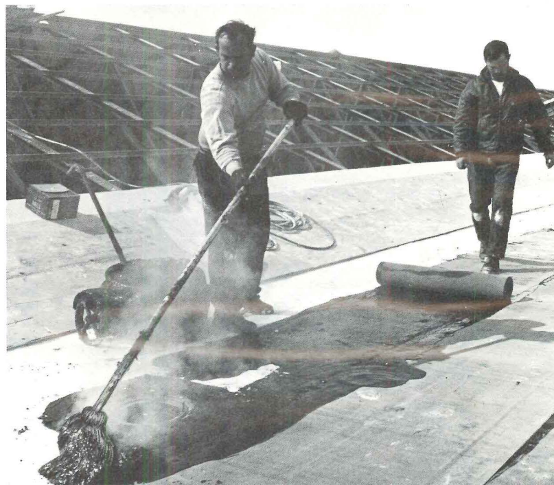
4 Tough, rigid polyurethane surface takes hot asphalt adhesives in stride, supports normal roof loads.
