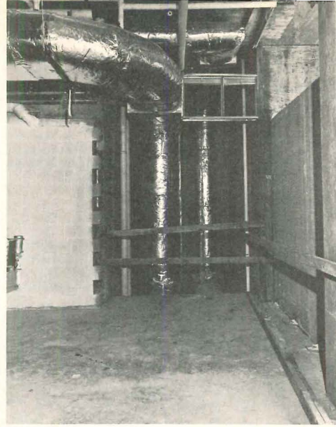
The complete sequence of utility distribution is shown in the photos. From left, clockwise: 1) horizontal mains at the lower level; 2) supply ducts and pipes emerging from one of the mechanical service towers, and turning down the corridor; 3) branch mains in a corridor, with stub ducts penetrating corridor masonry wall; 4) above ceiling space in one of the laboratory modules, showing reheat boxes, branch ductwork, piping, and conduit; 5) exhaust ducts at the roof; 6) fan-coil ducts at perimeter.
