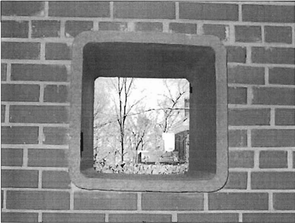
Detail of East Interior Wall of Carport
