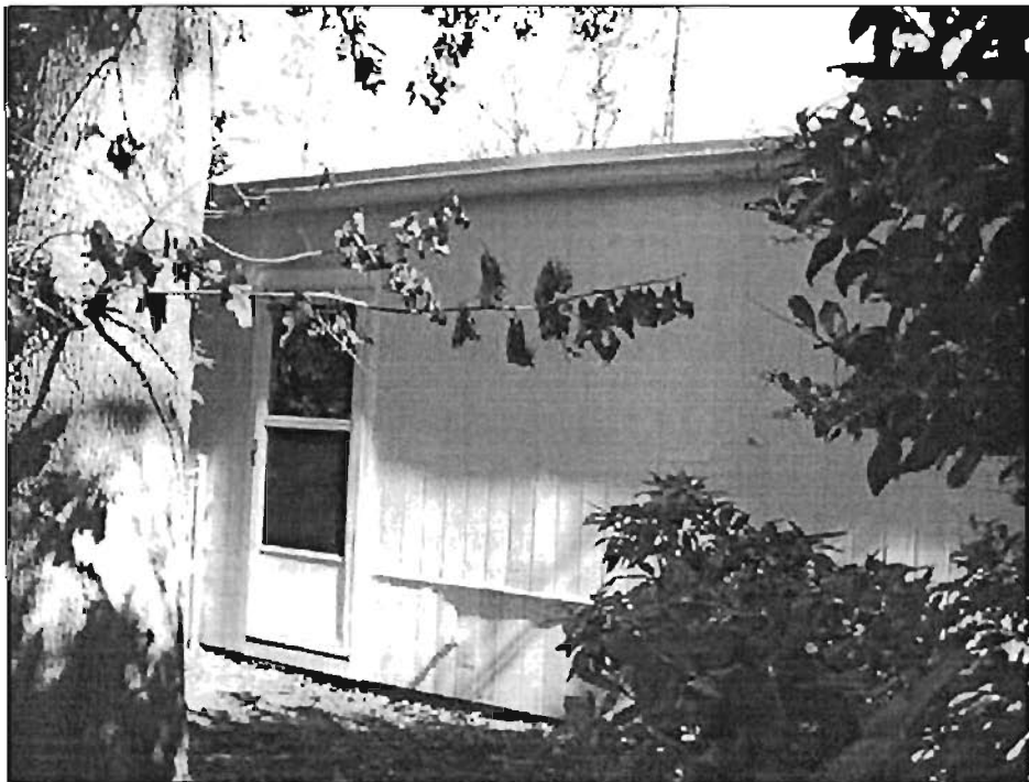
West Elevation (siding detail)
