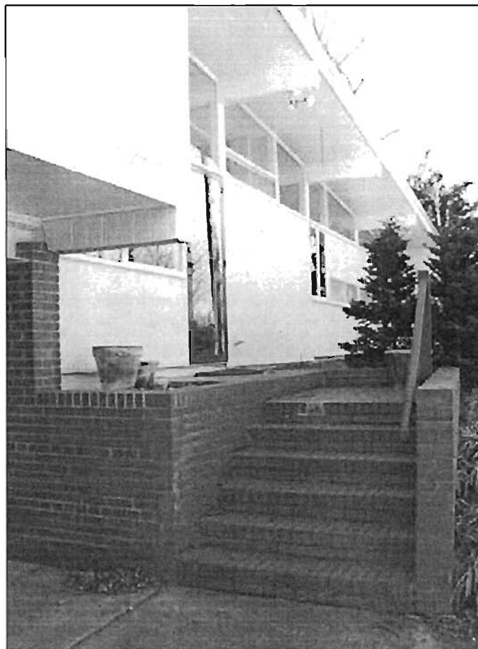
Front Entry Stairs
