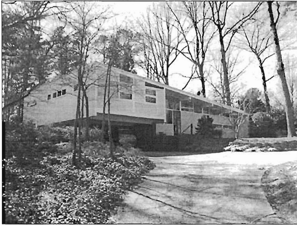
Façade/North Elevation (view of northeast corner)
