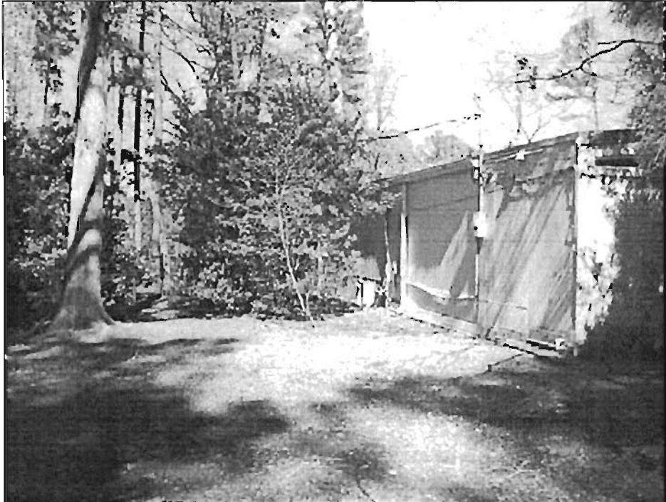
West Elevation (looking north)
