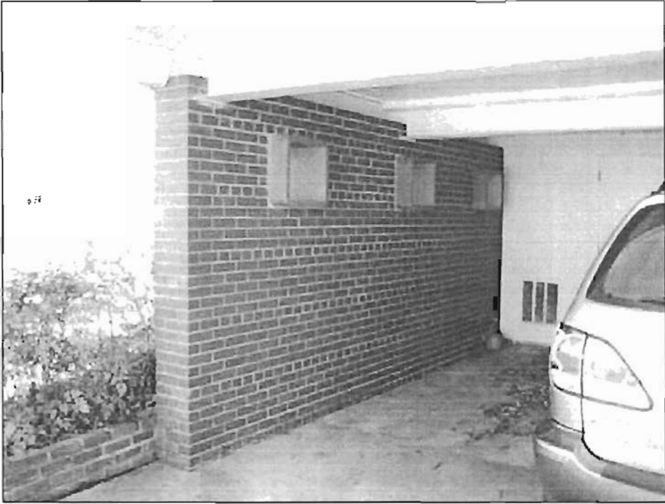
East Interior Wall of Carport
