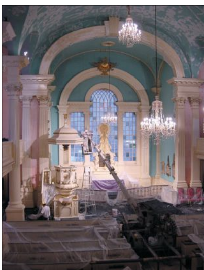
John Tiedemann used a boom system when restoring the decorative painting at St. Paul's Chapel in New York City.
