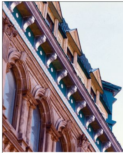
This stamped sheet-metal cornice was fabricated by W.F. Norman.
