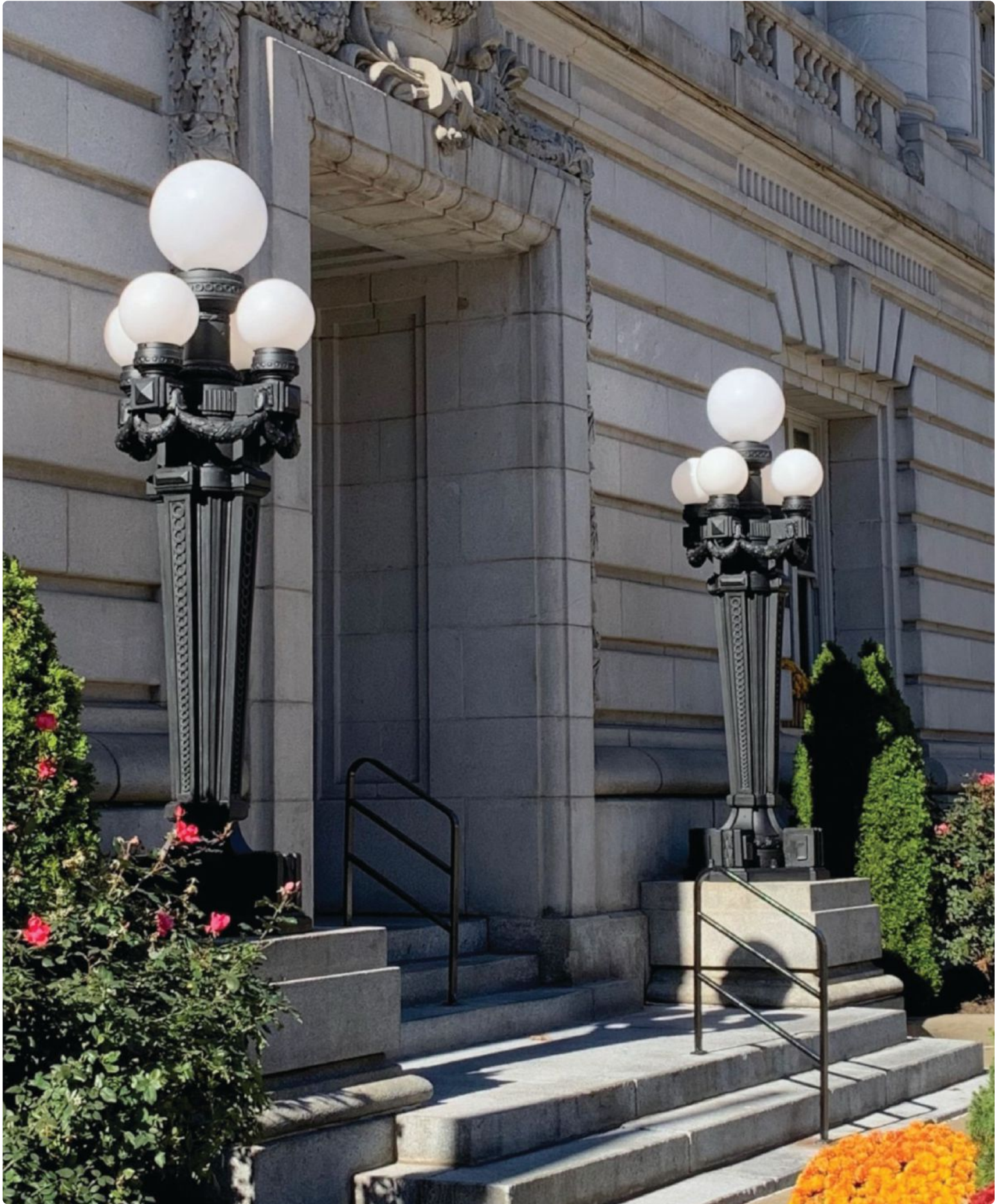
Lighting Restoration - Wheeling, West Virginia Courthouse
