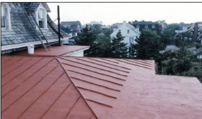
This metal roof has been treated with a waterproofing, elastomeric Acrymax coating from Preservation Products .
