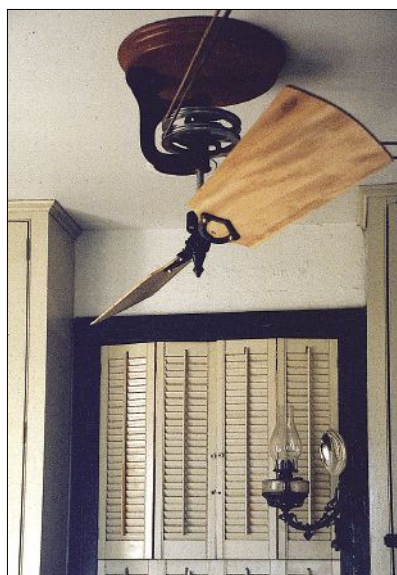
This belt-driven ceiling fan with solid-mahogany blades was supplied by Woolen Mill .
