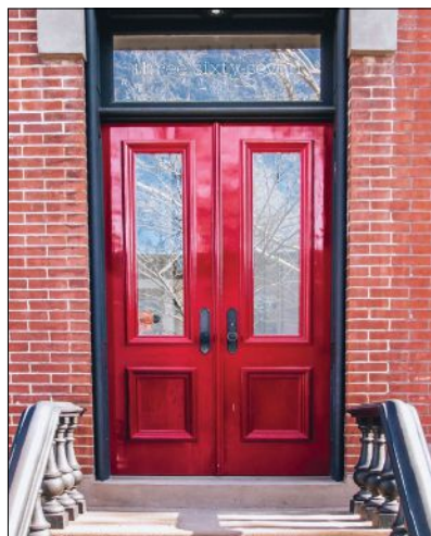
These vibrant red glazed and paneled doors were commissioned to replace a single door with a double-leafed entry doors on a 1880's Park Slope brick row-house by Brownstone Doors .
