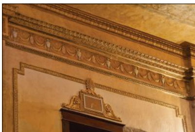
This historic plaster was restored by Swiatek Studios .
