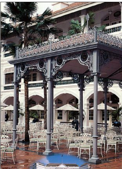
This intricate canopy with cresting and columns was custom fabricated by Robinson Iron Corp. for the Raffles Hotel in Singapore.
