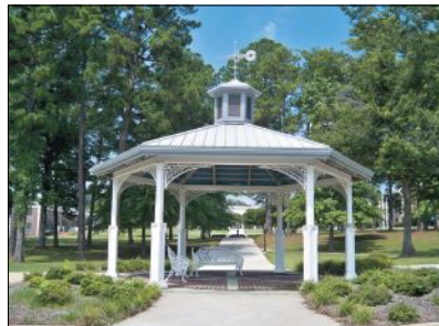
Robinson Iron designed and installed this custom gazebo of cast iron and fabricated waterjet-cut steel for the Central Alabama Community College in Alexander, City, AL.
