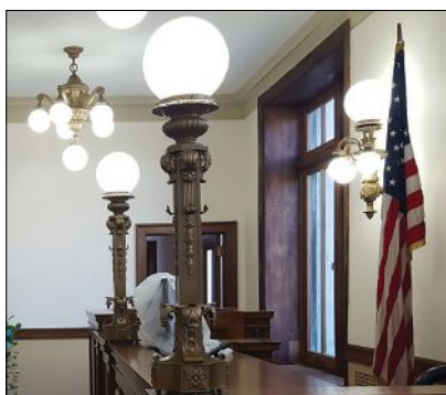
Grand Light provided the chandeliers, wall sconces and torchieres for the Hudson County Courthouse in Jersey City, NJ.
