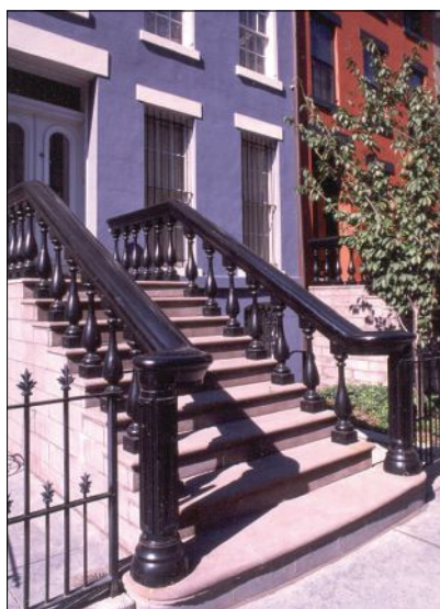
These traditionally styled balustrades were fabricated for a building in Brooklyn, NY, by Allen Architectural Metals .
