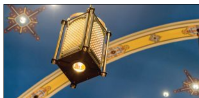
In designing and renovating the interior of Cathedral of Our Lady of Perpetual Help, Oklahoma City, Rambusch planned, built and installed a scene-controlled lighting system, incorporating both engineered and decorative LED fixtures. All lighting fixtures were manufactured in Rambusch's New Jersey workshops. Additional features included furnishings — altar, ambo, reredos and cathedra — with a side oratory honoring the Blessed Stanley Rother.
