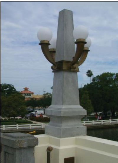
This decorative exterior lighting fixture was fabricated by Allen Architectural Metals for the Platt Street Bridge in Tampa, FL.
