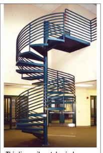
This line-rail metal spiral staircase was designed and manufactured by Stairways.
