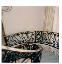
This forged-iron railing and polished-bronze cap rail were designed, fabricated, finished and installed by Wiemann Metalcraft.
