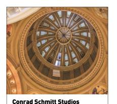
removed, conserved, re-leaded and reinstalled the stained-glass of the South Dakota State Capitol; the glass in the rotunda dome and the glass in the barrel-vaulted ceiling went through the extensive conservation process.
