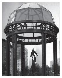
**Robinson Iron** fabricated the Woodruff Pavilion in Olympic Park, Atlanta, GA; it features cast columns topped with a transparent glass dome on a steel frame.
