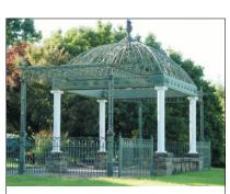
Wiemann Metalcraft fabricated this gazebo, fence and trellis in cast and wrought iron.
