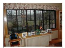
Interior glass storm windows from Innerglass Window Systems were used in this room.
