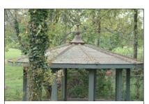
This gazebo features W.F. Norman Corp.'s style A shingles with its continuous hip finish and a custom-made finial on top.
