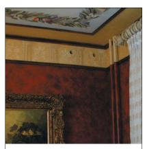
Unico's small-duct, highvelocity HVAC system takes up less than a quarter of the space of a traditional system, making it ideal for historic buildings.
