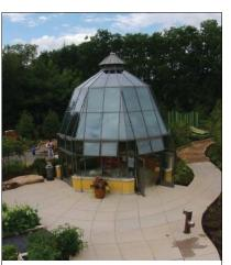
This octagonal greenhouse, fabricated by Glass House, features a custom color powder coat finish, power vented cupola, French doors and high performance glass.
