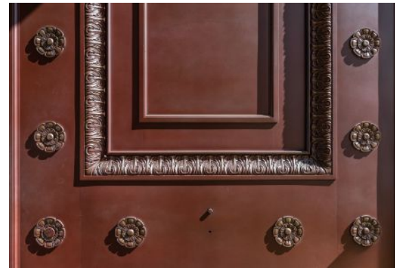
Several original bronze exterior doors had been replaced in years past. New doors were perfectly reproduced in bronze to match an existing original pair (left).
