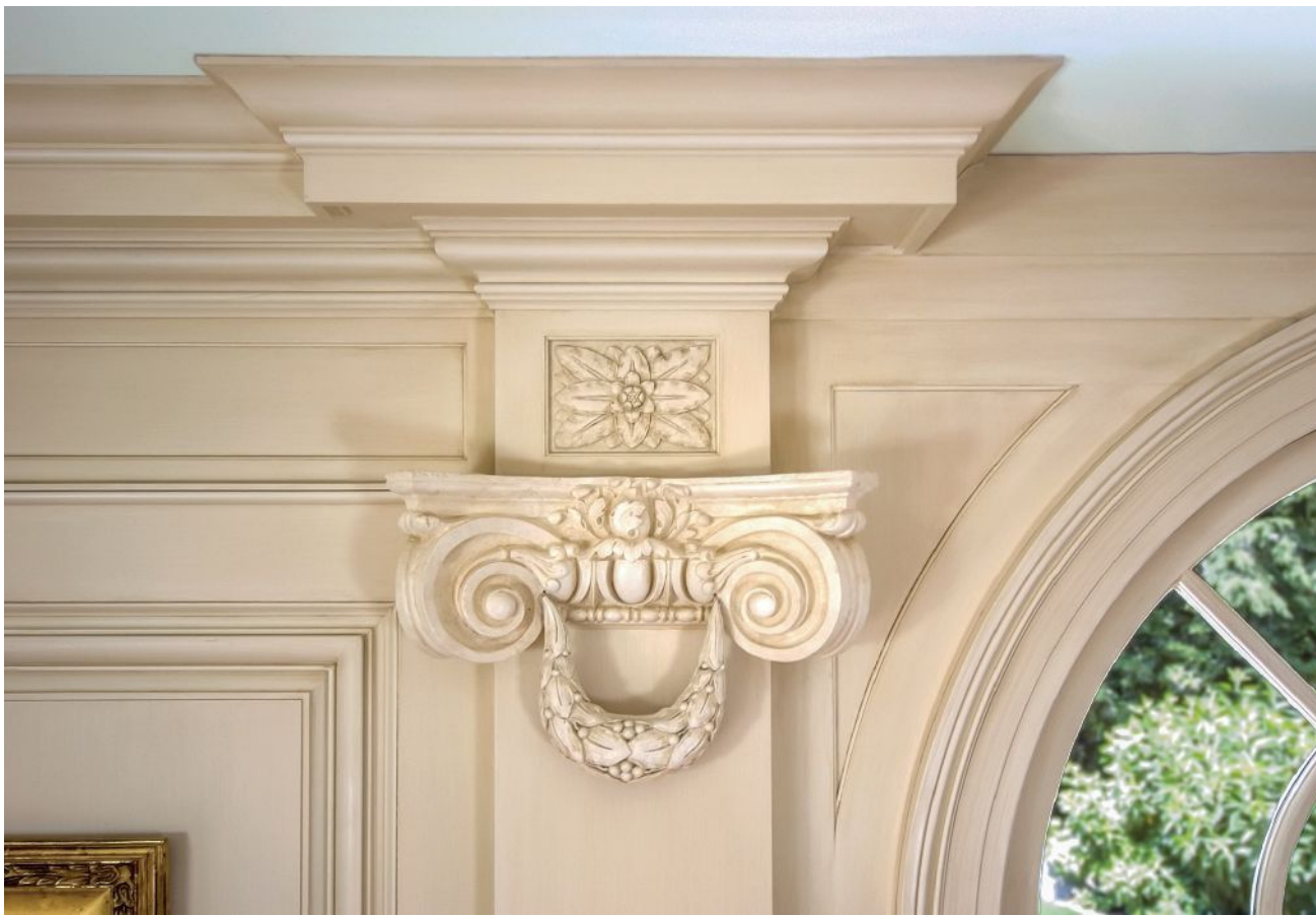
The adaptation of the Ionic order to the room by the elimination of the frieze was required by the height of the existing transoms over the French doors on the east and west walls of the room.
