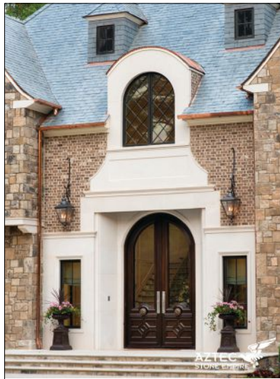
Aztec Stone Empire provided the limestone for this entrance.
