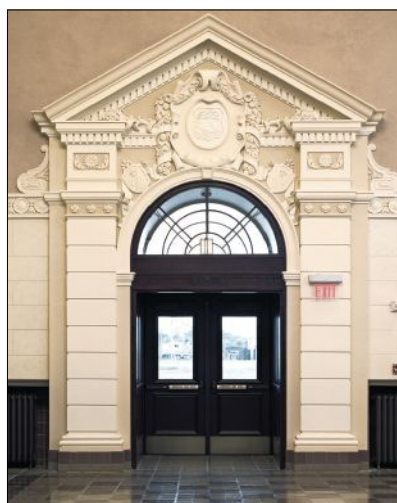
EverGreene Architectural Arts re-created the entrance to the Great Overland Train Station in Topeka, KS.
