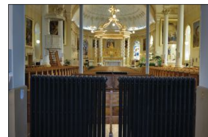
Shown here is a restoration of cast iron radiators in a church by Ecorad .
