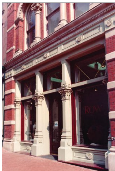
Historical Arts & Casting created these cast iron columns.
