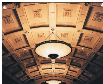
Flex Moulding used polyester resin to create this ornate bar-rel-vaulted ceiling.
