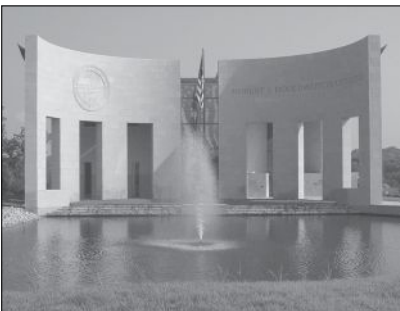
Continental Cast Stone created this stone monument for the Dole Institute of Politics in Lawrence, KS; the 14-ft.-dia. cast-stone medallion incorporates images of a farmer and plow, buffalo, cabin and steamship, as well as the state motto.
