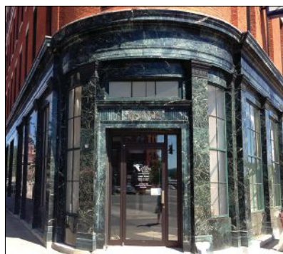
Vermont Verde provided the serpentine stone for this facade.
