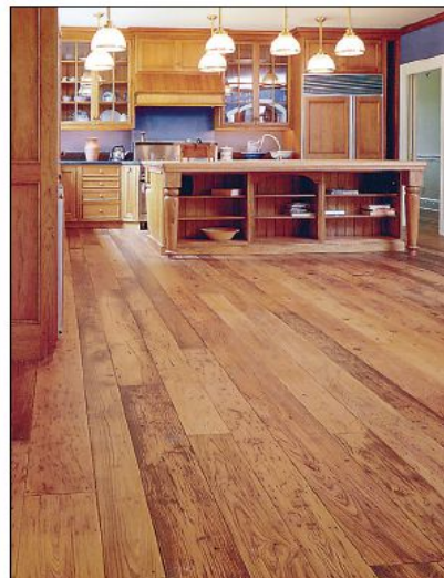
This random-width chestnut flooring was supplied by Chestnut Specialists and finished with oil and wax.
