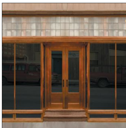
NIKO fabricated and installed the copper storefront and doors for this historic 1920s building in New York City.
