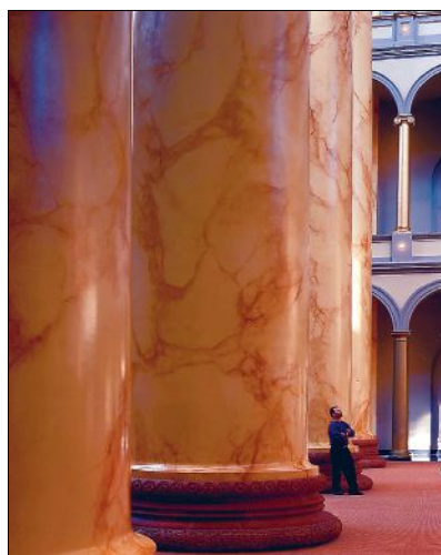
Canning Studios marbled these enormous columns in the National Building Museum in Washington, DC.
