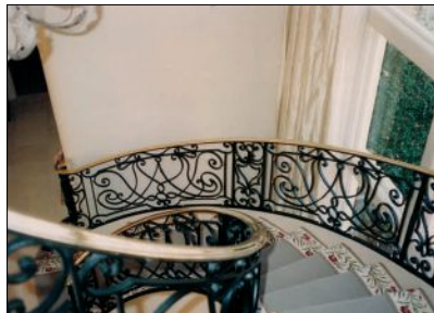
This forged-iron railing and polished-bronze cap rail were designed, fabricated, finished and installed by Wiemann Metalcraft .
