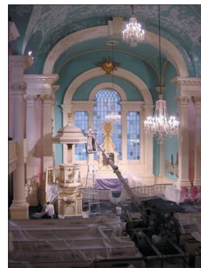
John Tiedemann used a boom system when restoring the decorative painting at St. Paul's Chapel in New York City.
