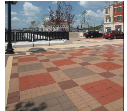
Paving from Belden Brick was used to create this decorative pattern.
