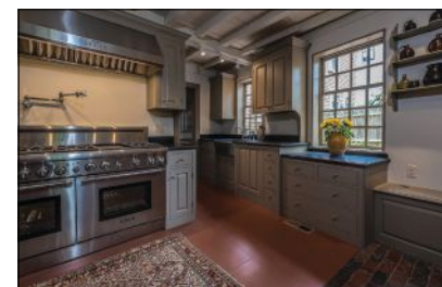
The Richard Holman house in Massachusetts was restored using cabinetry from Kennebec Co . Every cabinet was hand-crafted with hand-planed select New England pine and carefully fitted into the antique structure.
