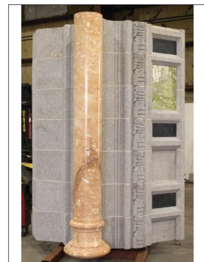
KEPCO+ attached three types of marble and Englishman Bay gray granite to a galvanized steel frame to create this detail.
