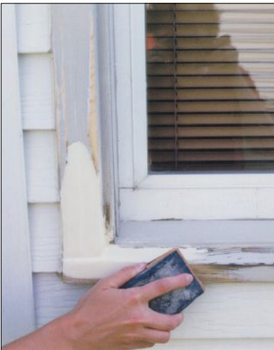
Abatron's LiquidWood restoration system regenerates and waterproofs dried out or spongy wood.
