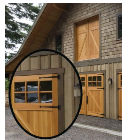
Richards-Wilcox butterbean hinge on carriage house doors feature their original design from 1880.
