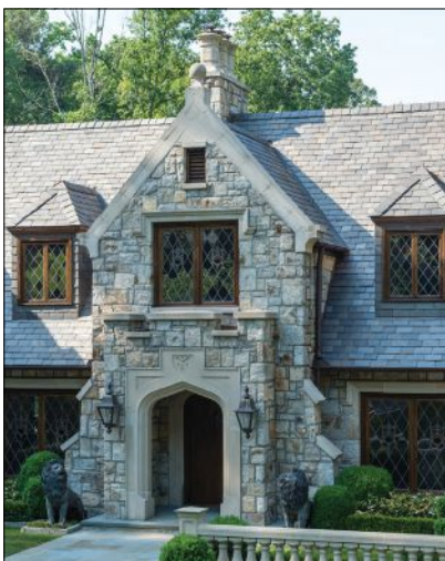
Aztec Stone Empire provided the weathered granite veneer and cut Indiana Buff Limestone accent details for this 2018 Palladio Award winning project.
