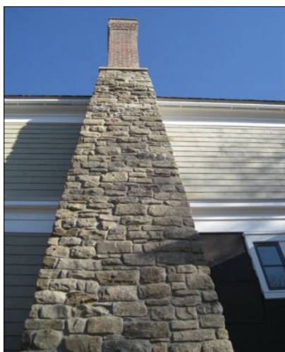
Reclaimed stone from a historic reservoir was paired with antique Purington Street pavers from Gavin for this chimney in Iowa City, Iowa.
