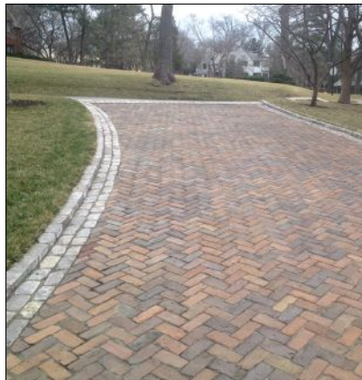
Gavin Historical Bricks supplied its reclaimed Purington Skinny street pavers and Antique European Blend granite cobblestone for this driveway in Kansas City, MO.
