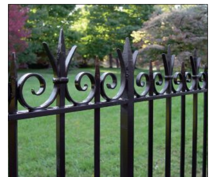
This custom fence was designed and fabricated by Wiemann Metalcraft using solid-bar steel; to ensure longevity, it was galvanized before urethane coating was applied.
