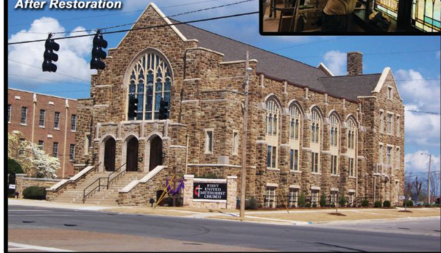
Before and after photos of the F4 tornado damage to the First United Methodist Church of Cullman, Alabama restored by Bovard Studio Inc
