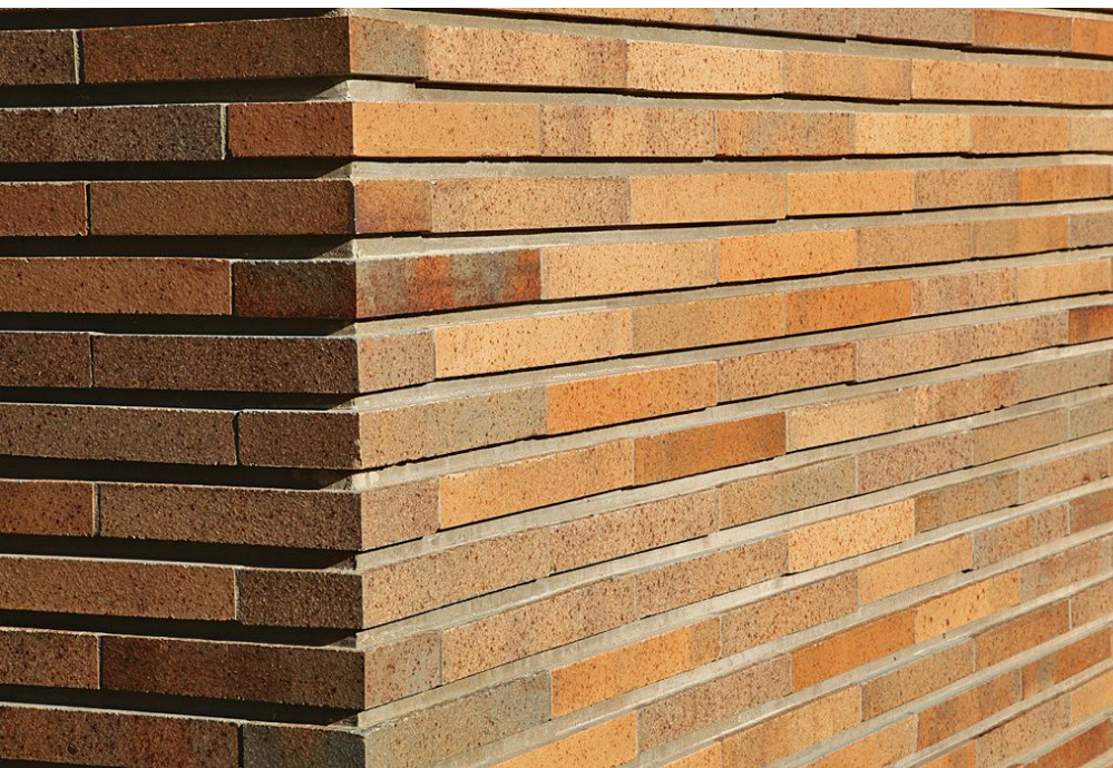
LEFT: The iron-spots bricks Belden Brick Co. made for Frank Lloyd Wright's Darwin D. Martin House Complex in Buffalo, NY, were a unique size: 12 in. long, 4 in. deep and 1 5/8 in. tall. Photos: Maguire
