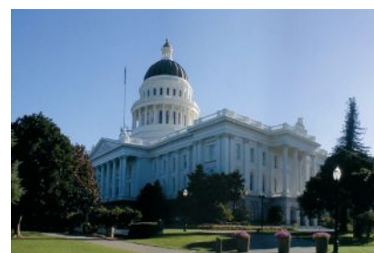
Avian Flyaway's bird-control system was installed on California State Capitol in Sacramento, CA.
