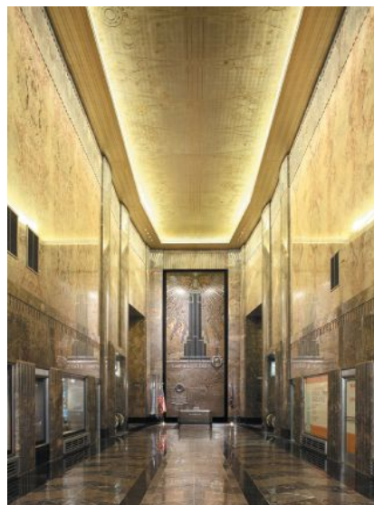
EverGreene re-created the aluminum and gold leaf ceiling mural in the lobby and hallways of the Empire State Building; work also included reinstating historic glass panels in the lobby, designed and cut based on historic plans and photographs.
