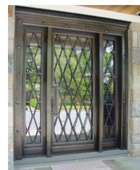
Wiemann Metalcraft fabricated this bronze door with insulated glass.
