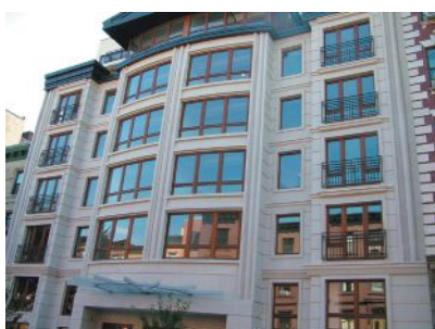
Haddonstone provided the custom cladding for this New York City building.
